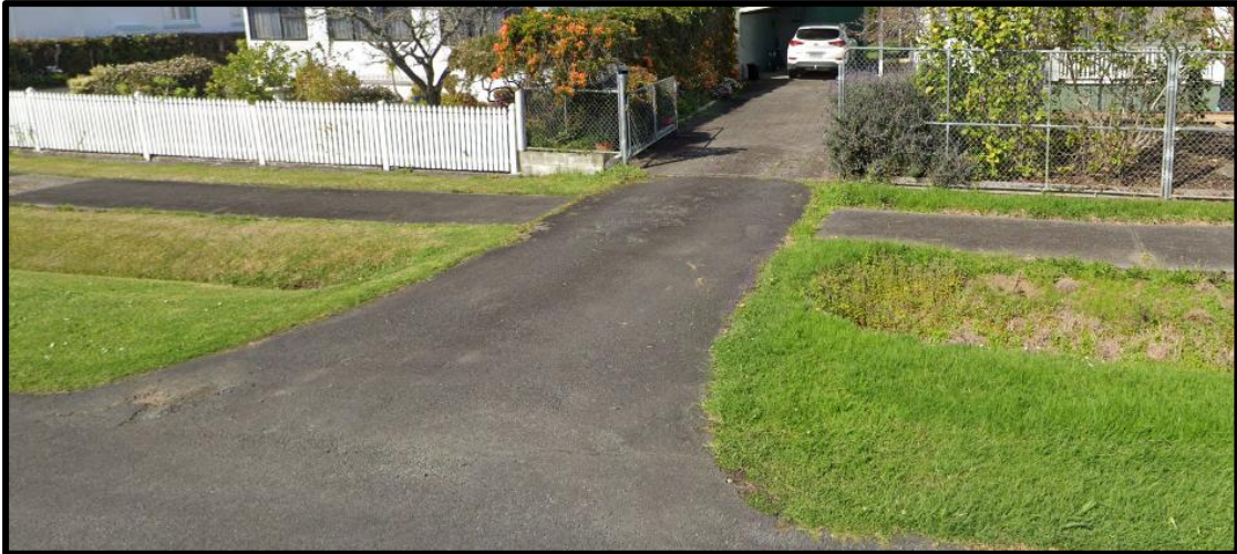
Figure 15: Existing sealed crossing and drive to Lot 1.
