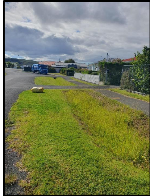
Figure 6: Image of the existing crossing and roadside drain to Lot 1.
