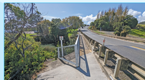
Upgraded handrails and adjoining paths make the bridge safer.
