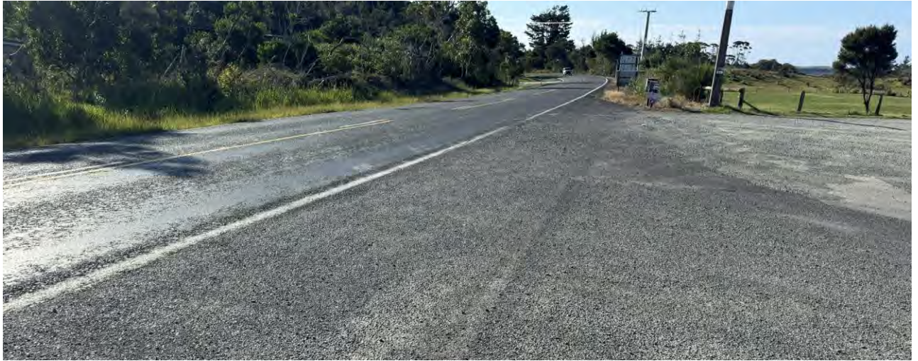
Photo 6. Looking north along Far North Road from the northern access crossing.
