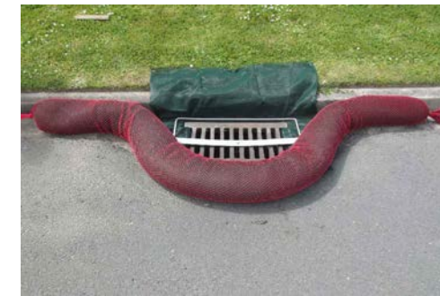
CATCH PIT E&S PROTECTION VIA SILT SOCK
