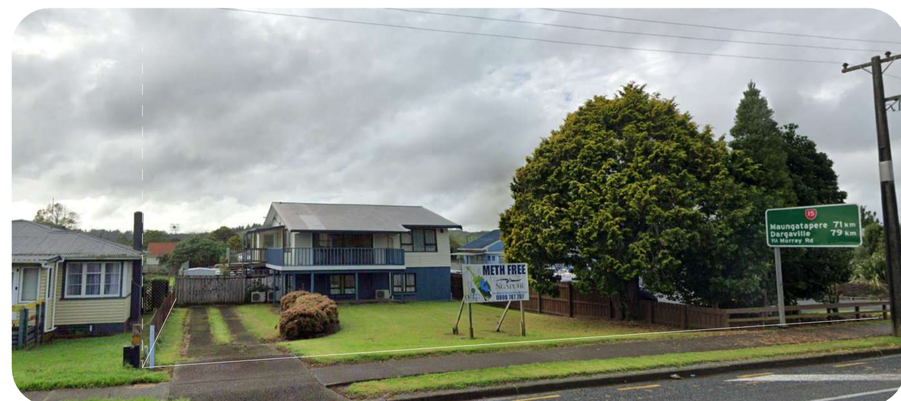
V1: Existing frontage of 12 (left) and 14 Mangakahia Road (right) looking North East. There is one vehicle crossing located along the western boundary, with a low steel mesh fence separating it from the neighbor property. The boundary fence adjoining 14 Mangakahia Road is a high timber fence with a low section at the front.
