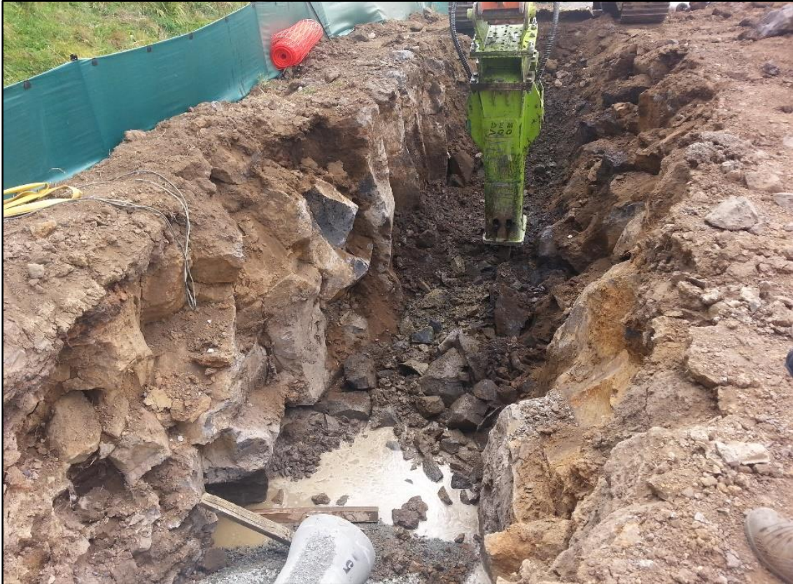
Heavy Duty Rock Breaking to Install Public Services
