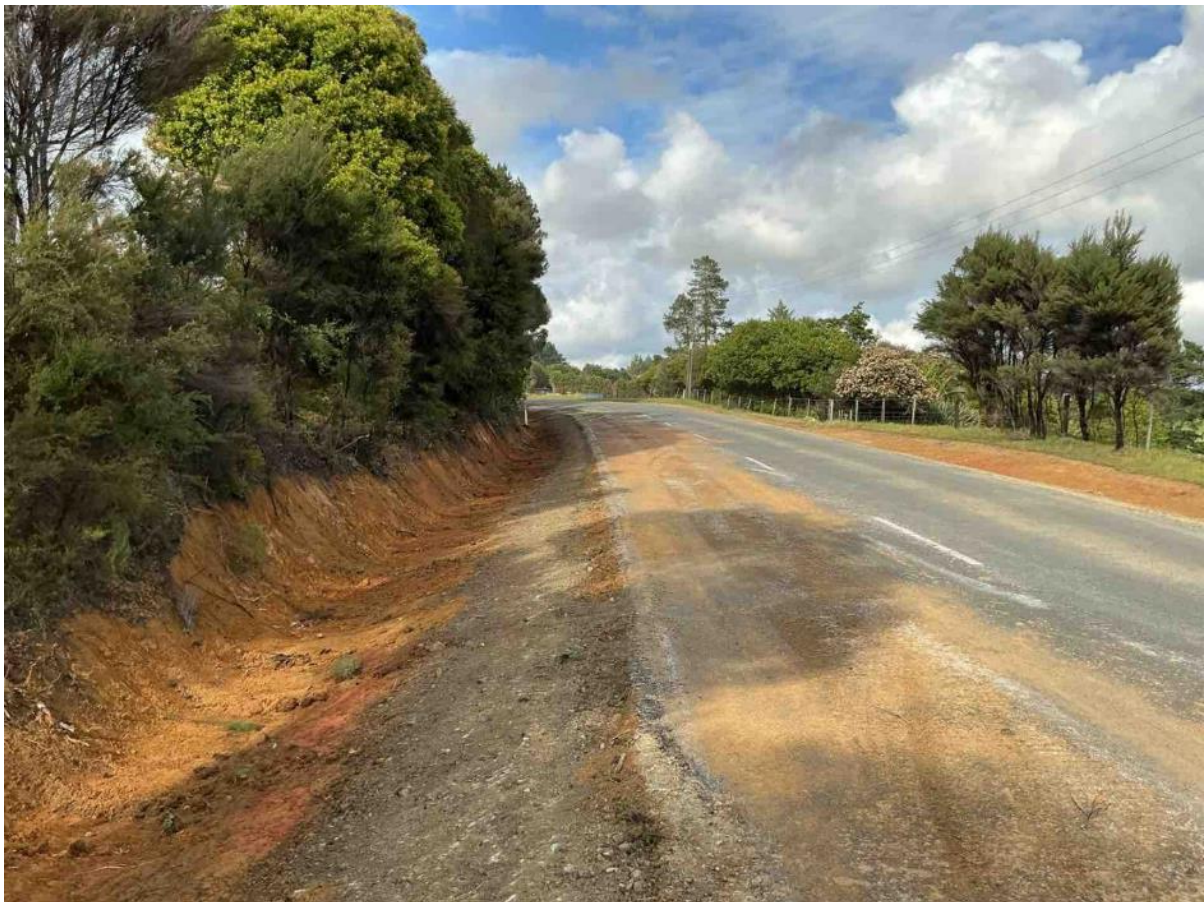
Site clearing – Hihi Rd Pavement Rehabilitation
