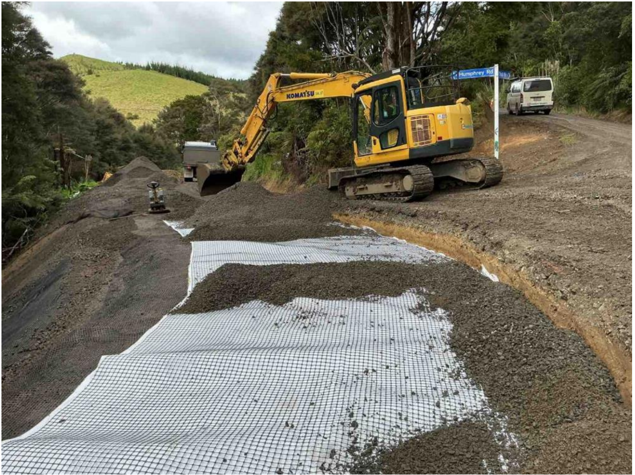
Humpfreys Rd – Slip repair in progress
