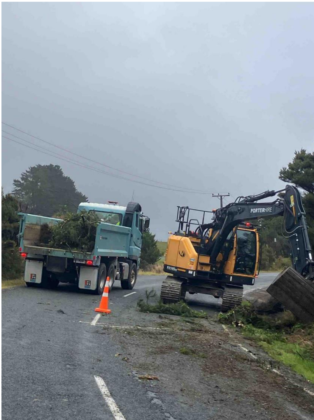
Hihi Rd Rehab – Site clearing
