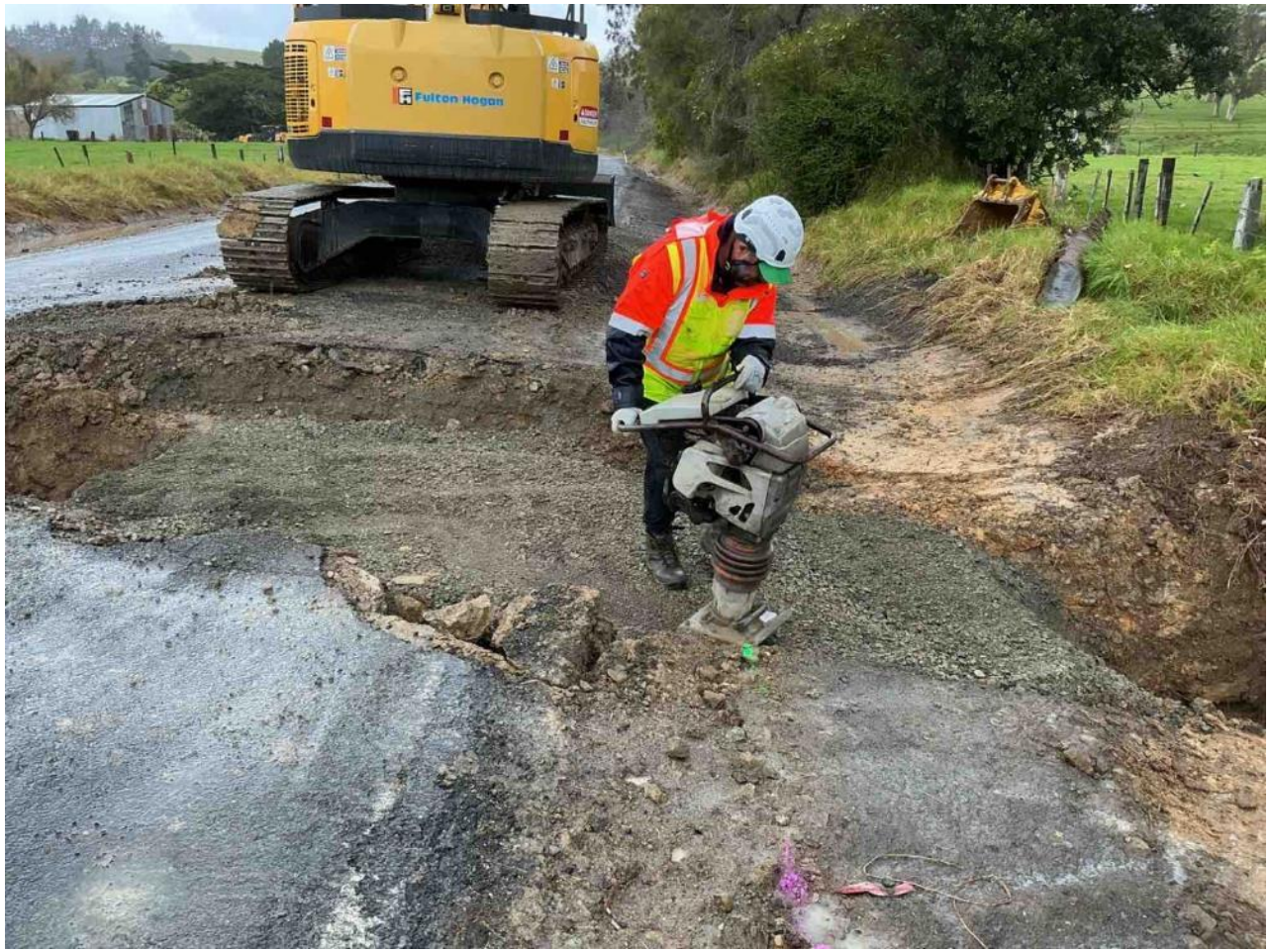
Hihi Rd Rehab – Drainage Renewals in Progress
