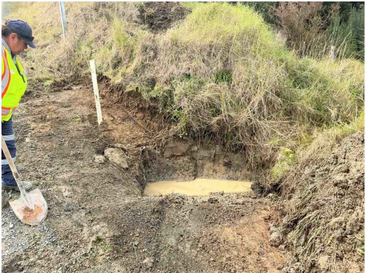
Culvert Clear Crew in action
