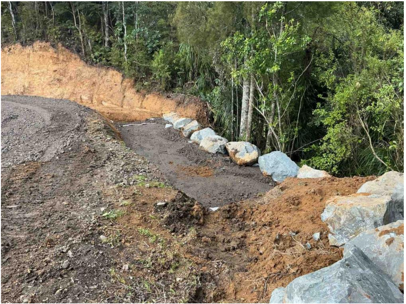
Humpfreys Rd – Slip repair in progress
