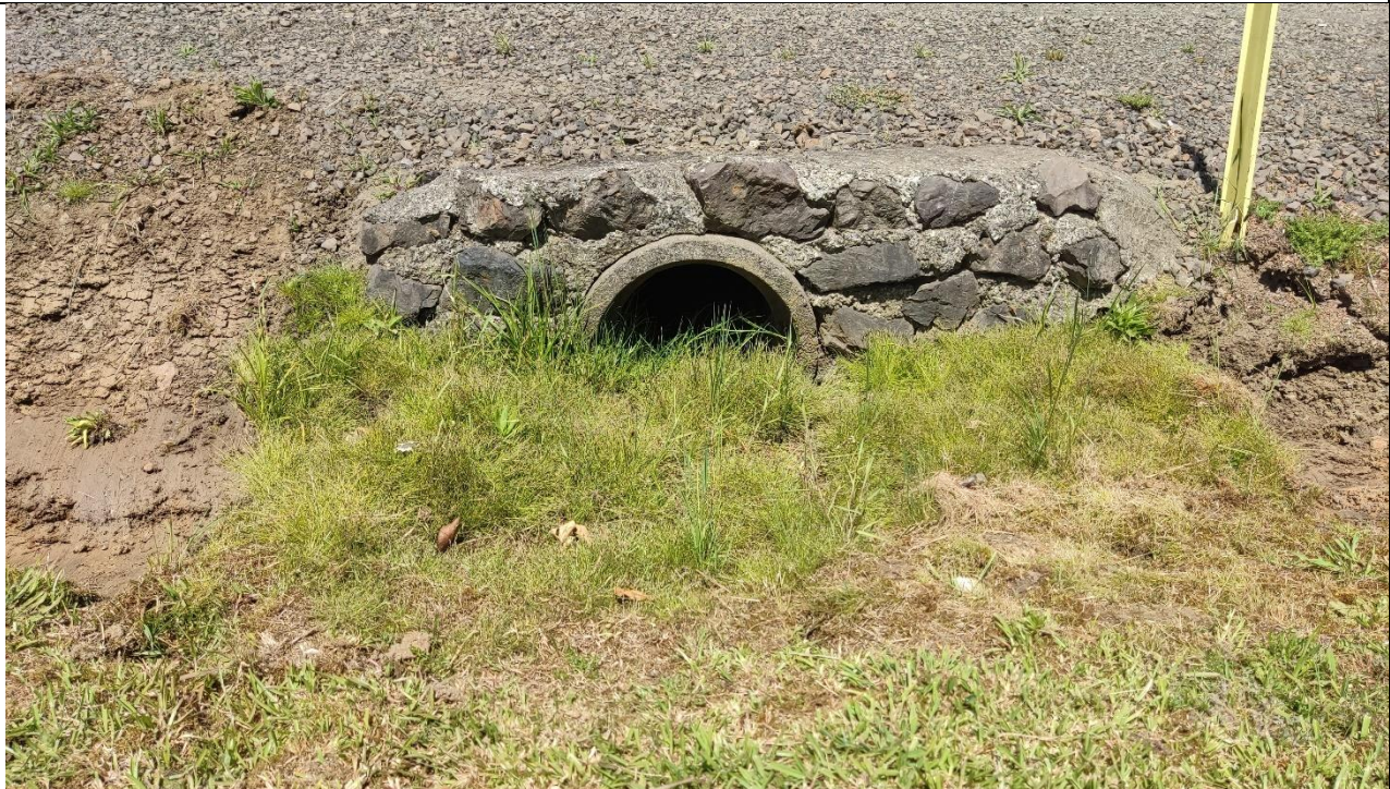
6. 375mm culvert under Wainui Road
