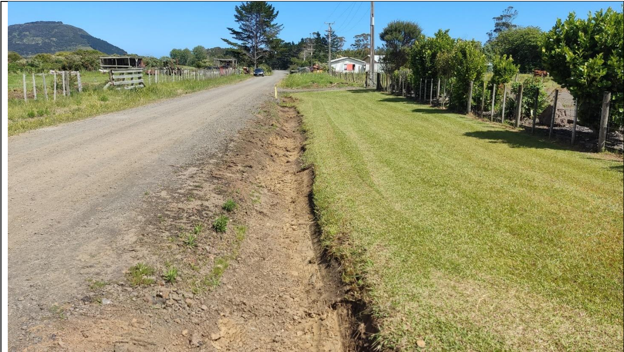
5. Roadside water table
