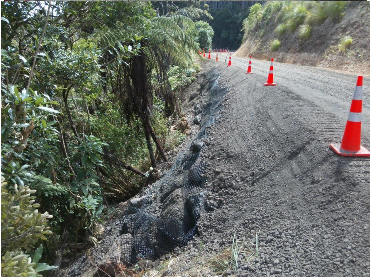
Completed Storm Damage Repair on Paponga Rd
