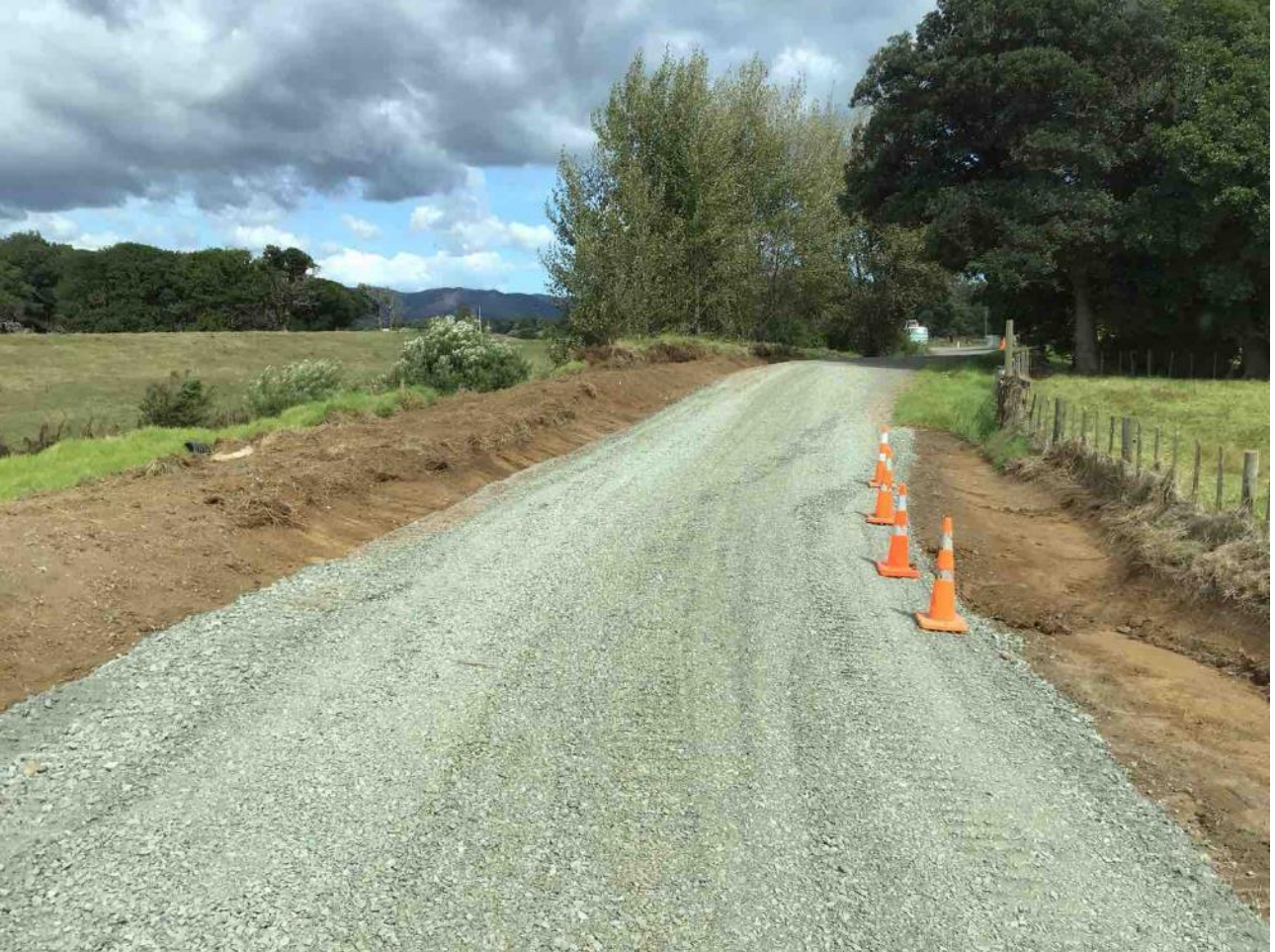
Completed Storm Damage Repairs on Duncan Rd
