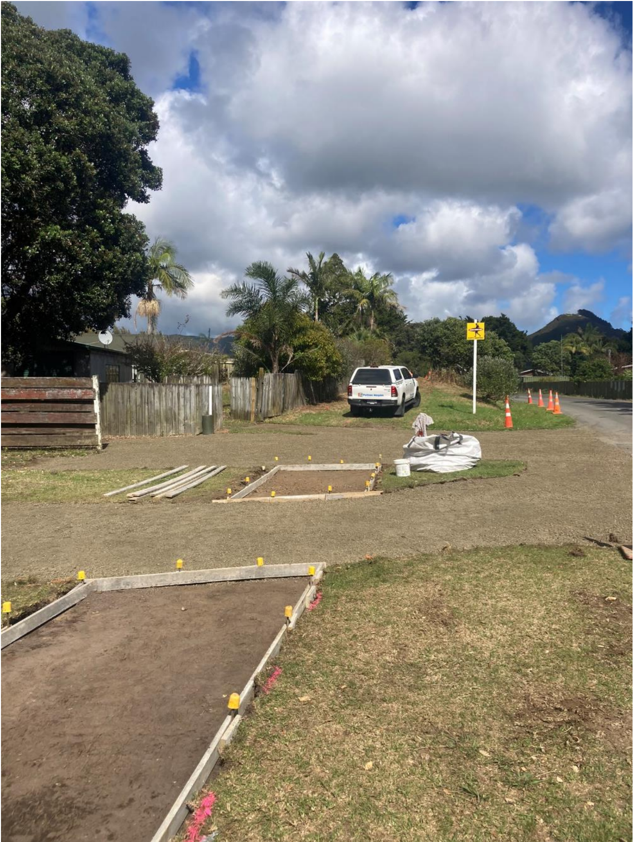
New Footpath in Construction Takaha Road Ahipara
