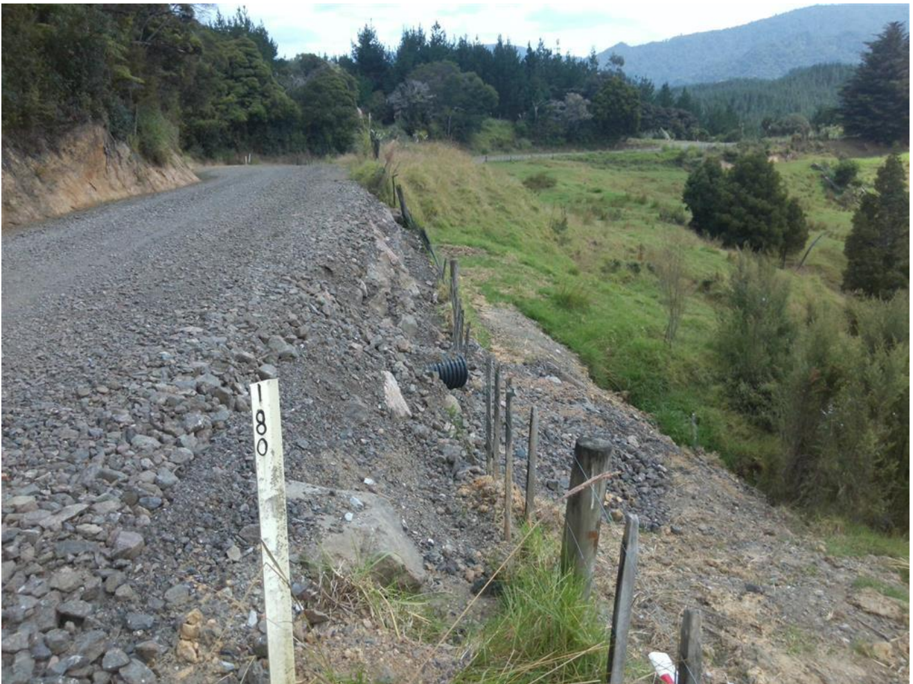
Storm Damage repair completed on Paponga Rd
