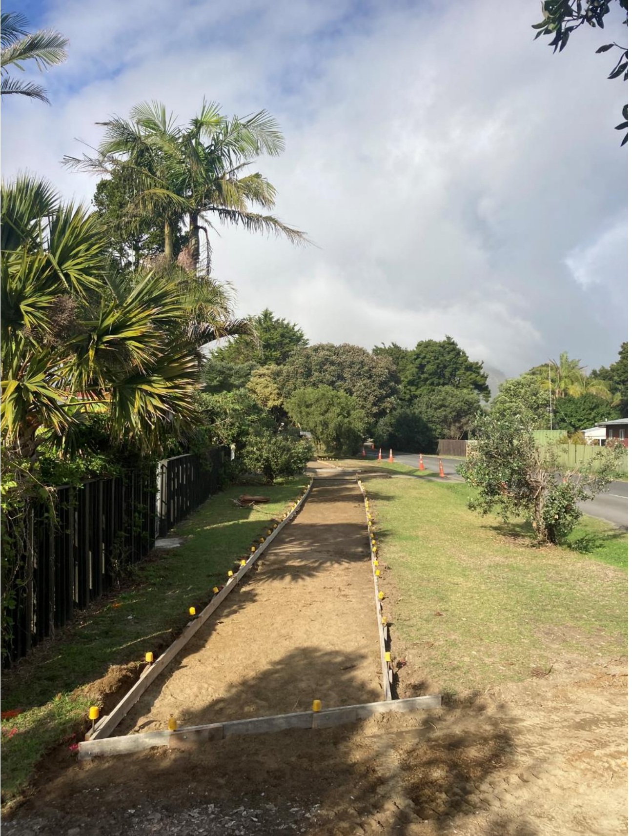
New Footpath in Construction Takahe Road Ahipara
