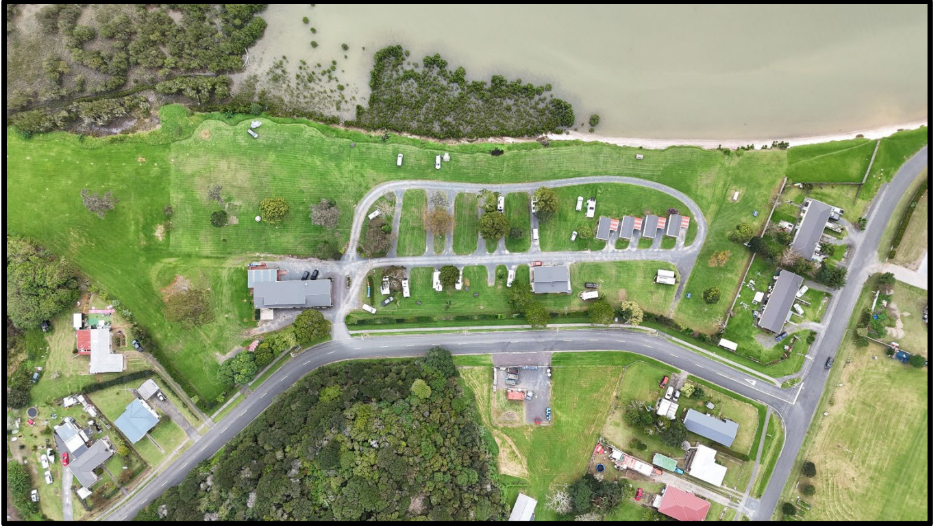
Photo 2: Aerial View of existing Waitangi Holiday Park
