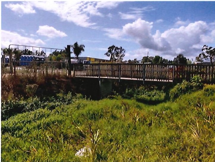
Figure 3 – Footbridge to remain
