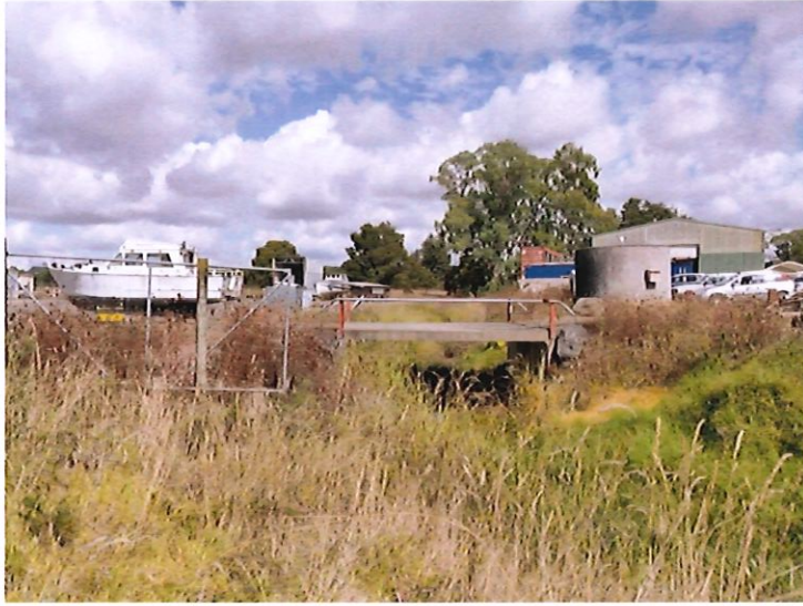
Figure 2 – Culvert to be removed
