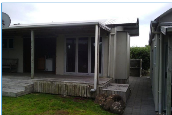
Photograph 1: Existing buildings on Lot 1. The water tank is located beneath deck.
