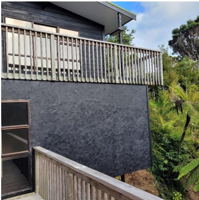
Edge of Sauna Room and Land Covenant Area B
