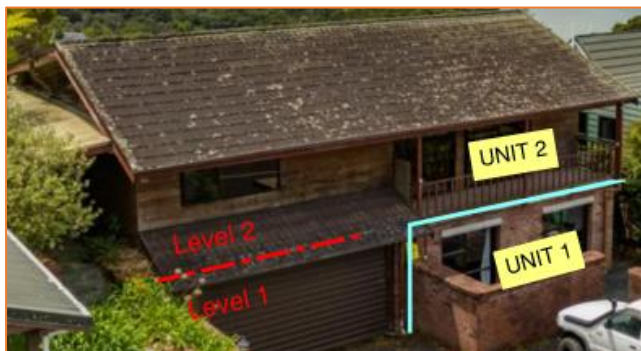
Figure 1: South Elevation (facing Te Haumi Drive)
