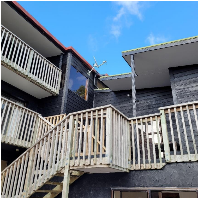
Common deck and staircase areas.
