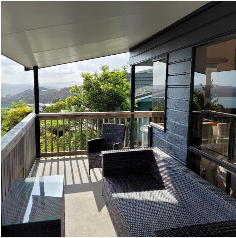
Upper Level (L1) deck of Area 2 (northern elevation)
