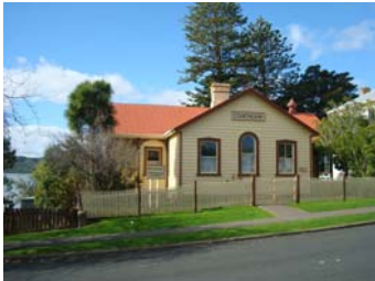
Former Court House
