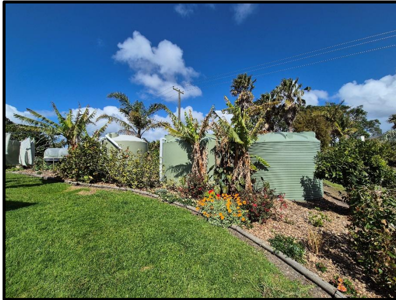
Figure 3: Existing water tanks on site. Tank on far right results in infringements of setback and sunlight given height of tank.
