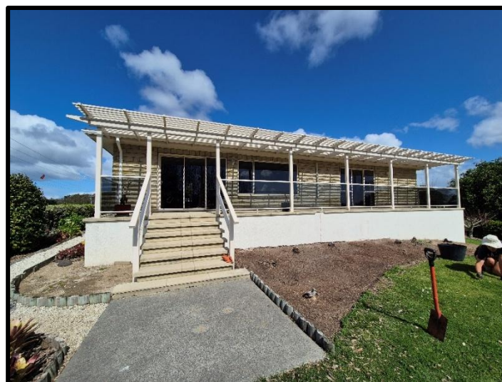
Figure 2: Deck to be replaced.
