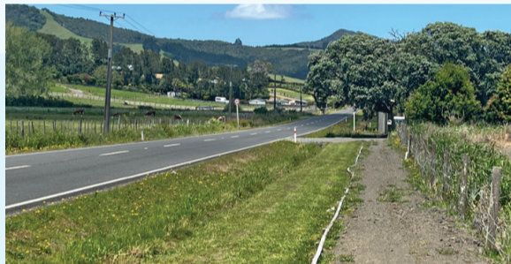
One of the new footpath locations along Kaitāia- Awaroa Road.
