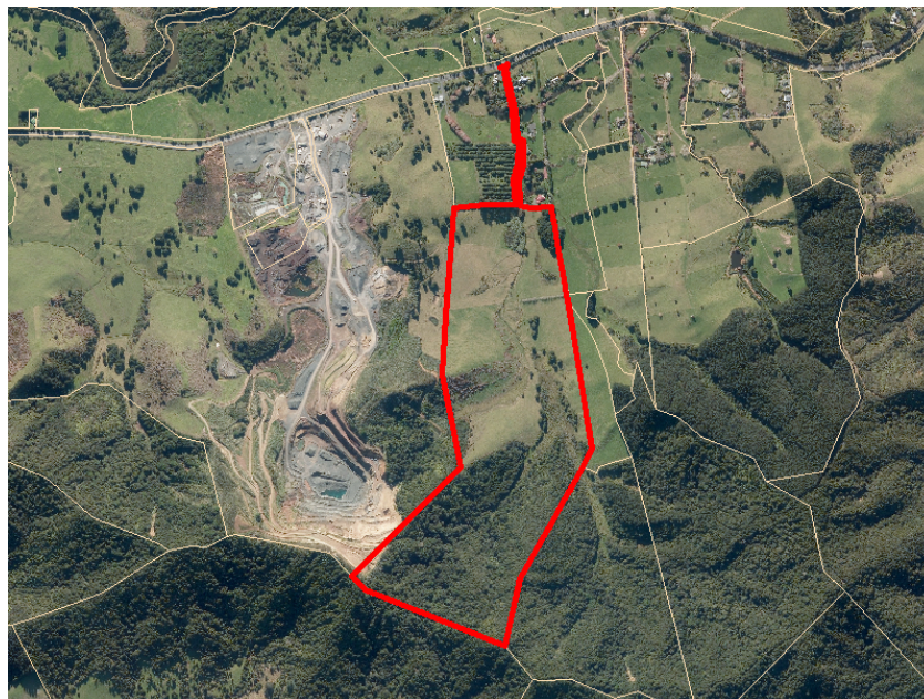
Figure 2 – Site RT NA97B/387 (Source: Prover)
