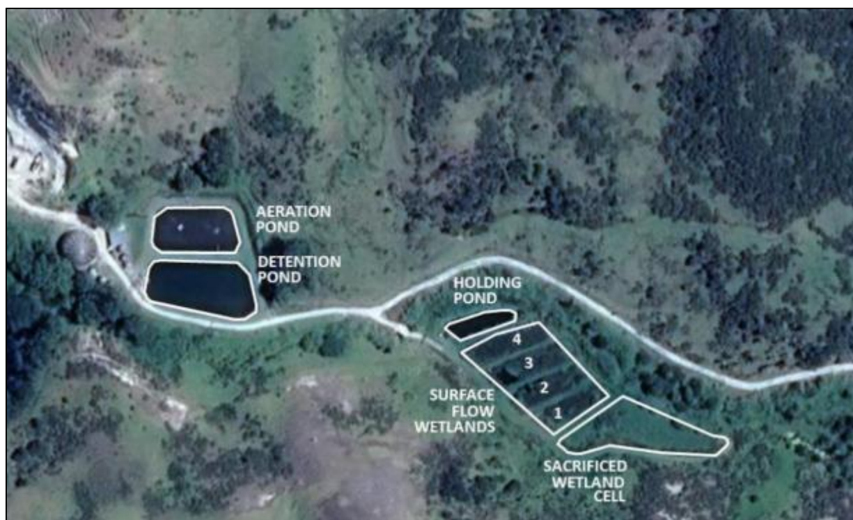
Figure 3-1: Aerial Photograph of Opononi WWTP
