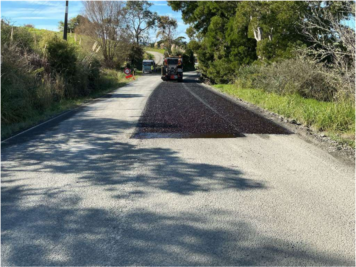
Fairburn Rd – Maintenance Pavement Repair with Jetmaster Seal
