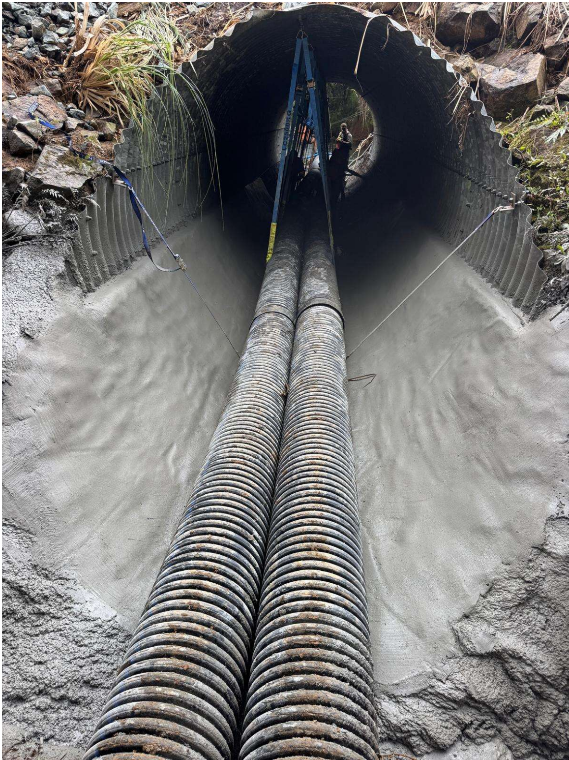
Kenana Rd – Culvert concrete lining (FNR)
