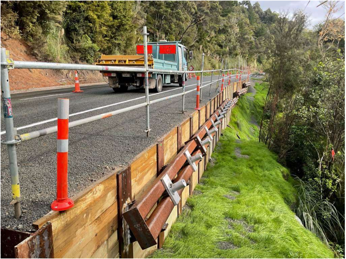
Mangamuka Rd Slip Repair (FH Civil)
