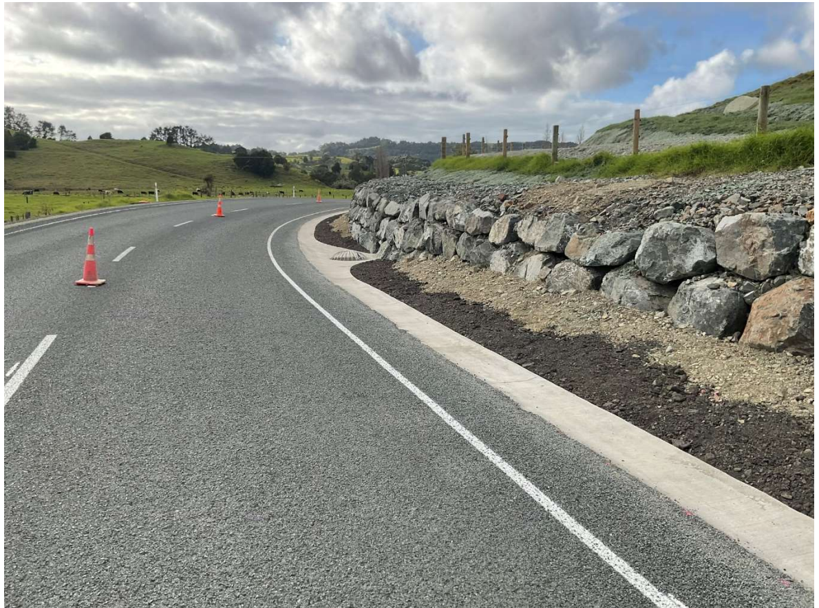
Fairburn Rd Rehab – Concrete Dish Channel (Sweetwater Construction)
