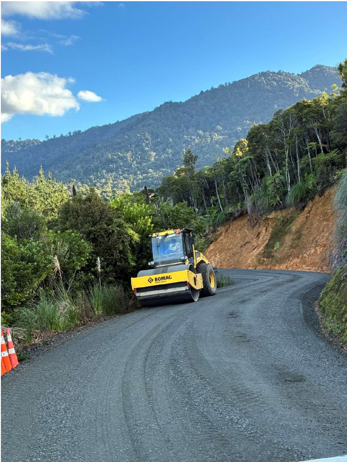
Paponga Rd – Unsealed Overlay in progress
