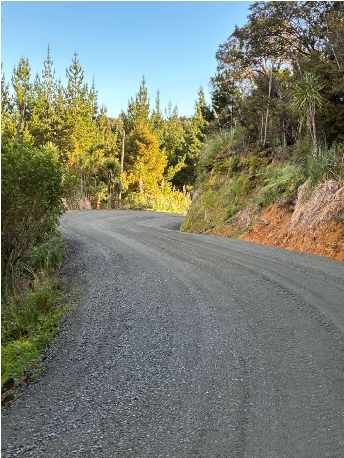
Paponga Rd – Unsealed Overlay in progress
