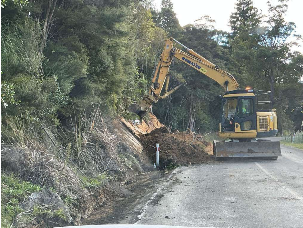
Broadwood Rd – Rehab Clearing
