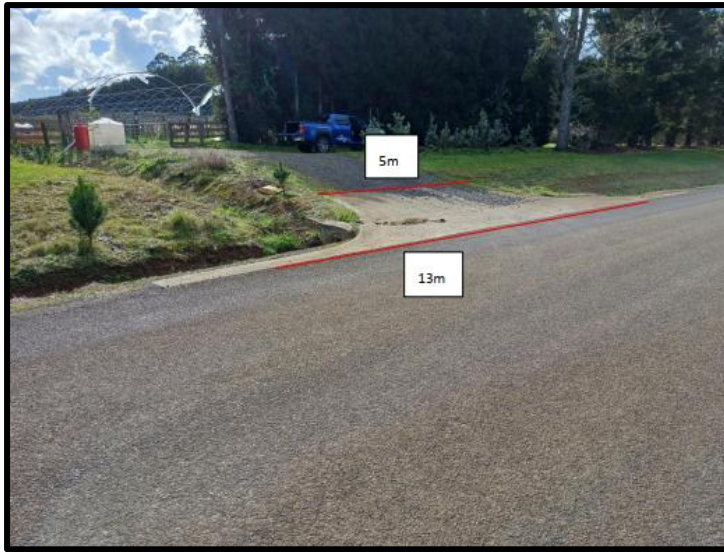
Figure 17: Existing crossing place to Lot 2 which has been determined to meet the required engineering standards.
