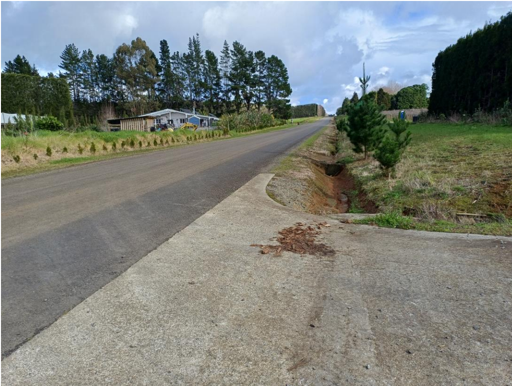
Figure 10 - Lot 2 existing vehicle crossing sight distance to west.
