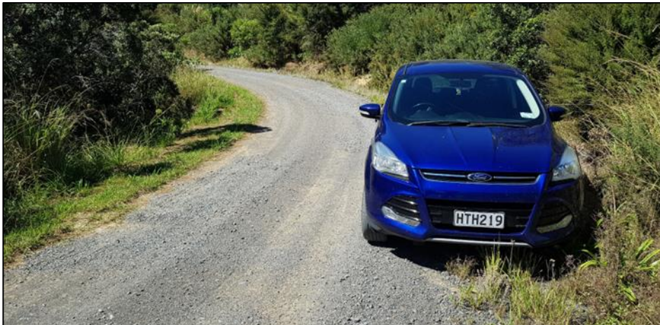
Corner at RP 580m looking northwards March 2022 (adequate width to widen carriageway to 5.5m on bend)
