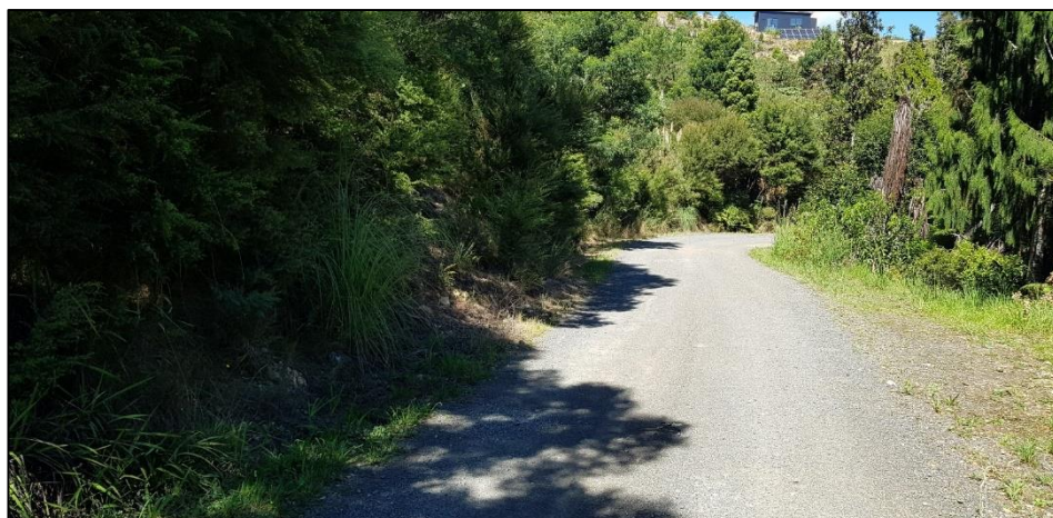
RP 800m looking southwards (adequate width for proposed passing bay prior to narrow section at RP830m)
