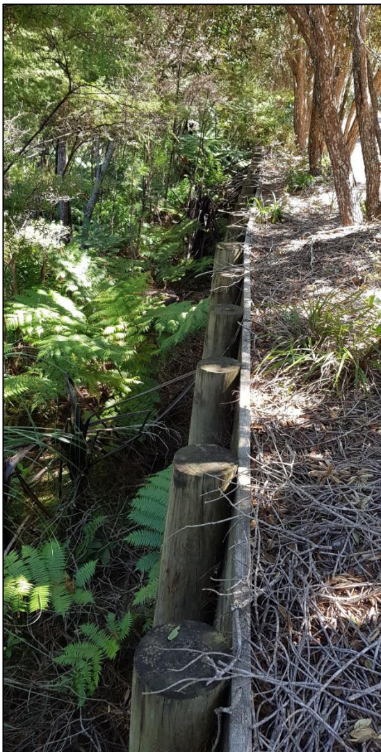
Timber Pole retaining RP 1010
