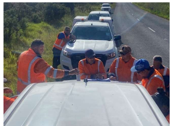
Ngapipito Rd – Pre commencement Korero.
