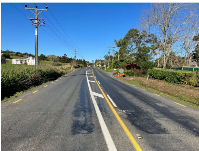
BEFORE Photo (Taken at Preseal Inspection)
