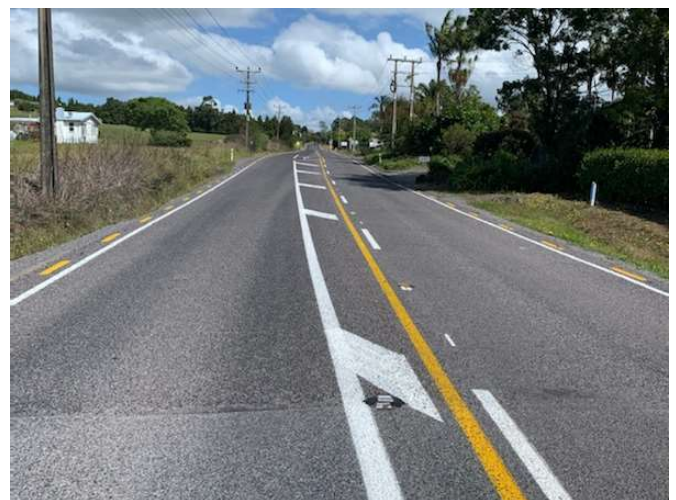
AFTER Photo (Taken after Resealing)
