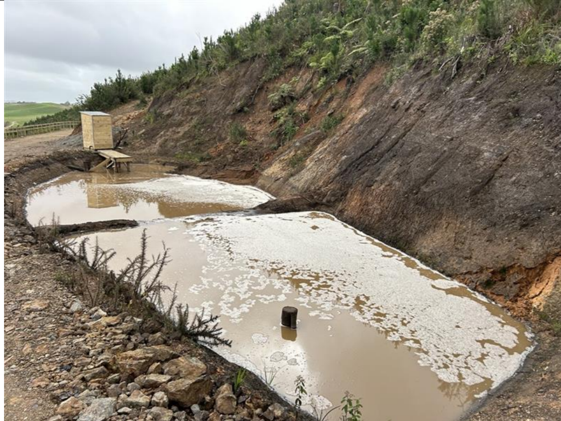
Photo 17: Northwest-facing view of the condensate pond.
