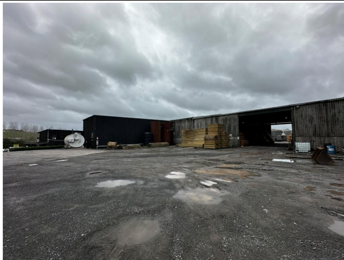
Photo 11: West-facing view of the AST storage yard.
