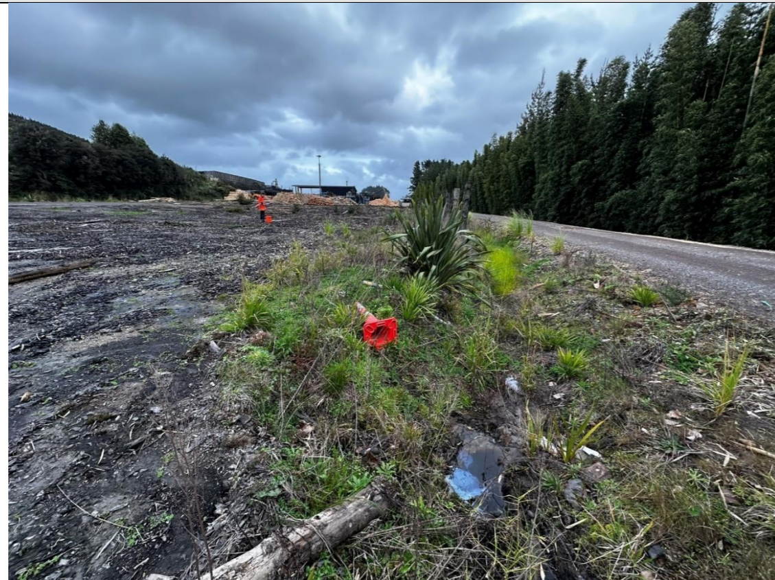
Photo 15: South-facing view of the raw timber storage yard. A small channel runs along the western side of the yard with an organic sheen visible on the surface of the water.
