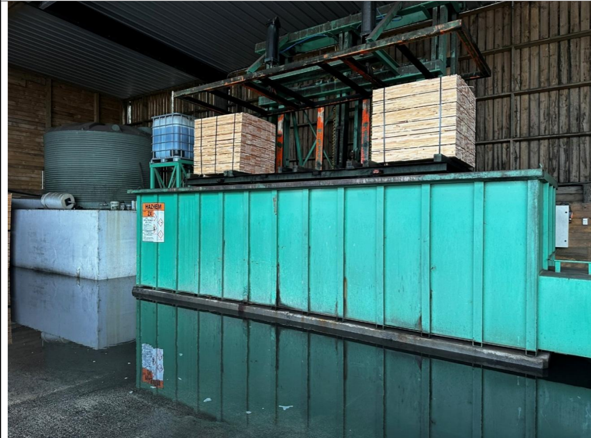
Photo 7: The dip tank where anti-sap treatment with Hylite NCF occurs. Liquid at the surface is rain water, entering due to the slope of the site,
