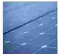
CF09 - SOLAR PANELS
