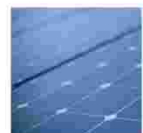
CF09 - SOLAR PANELS
