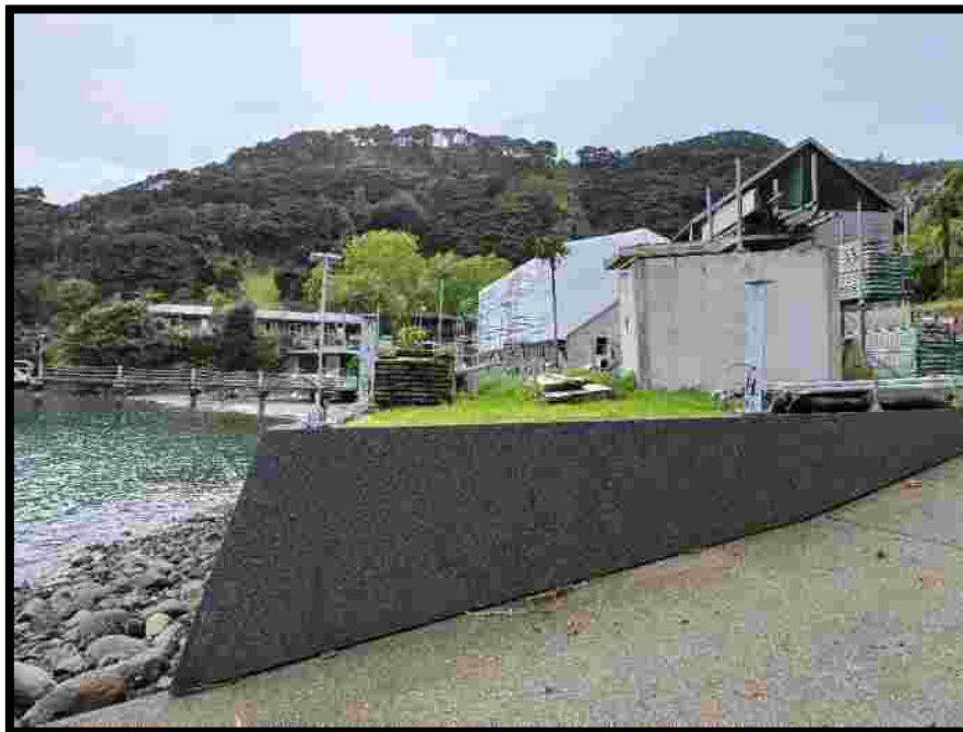
Figure 3 – Main lodge and boat shed currently under redevelopment
