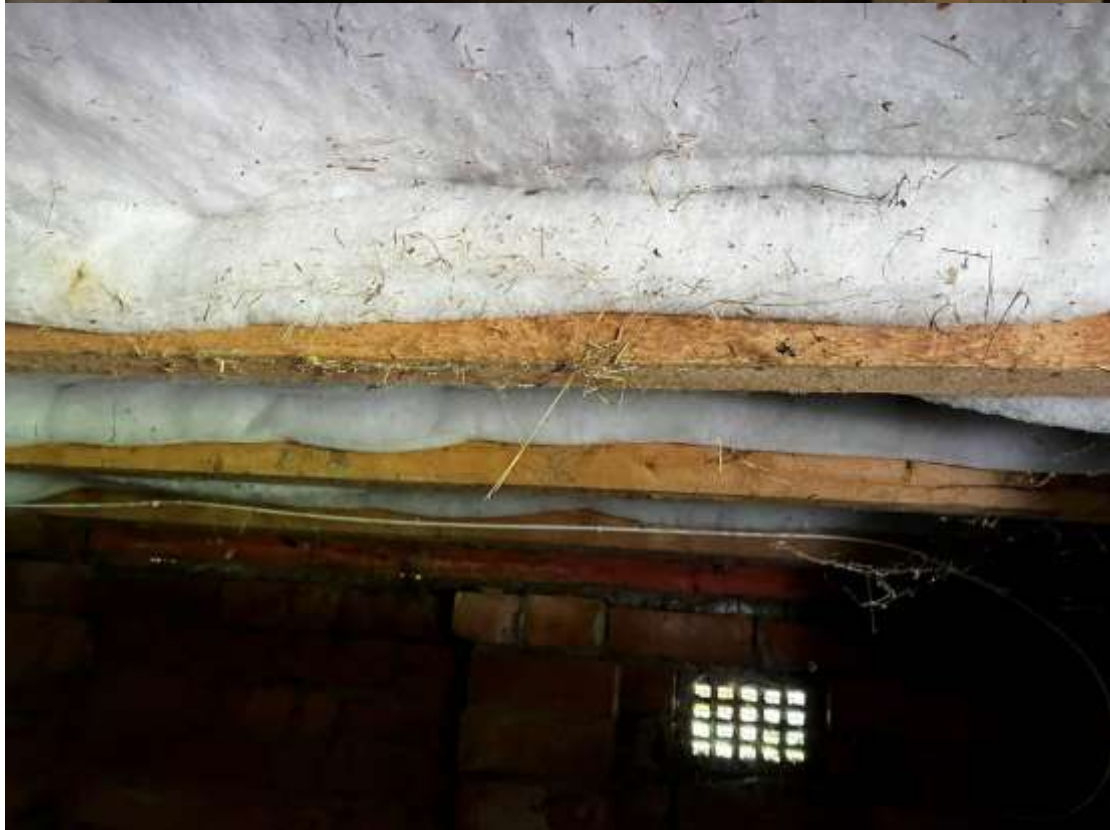
The ceiling space has 100x50mm trusses with purlins, an AV unit, building paper and insulation.
