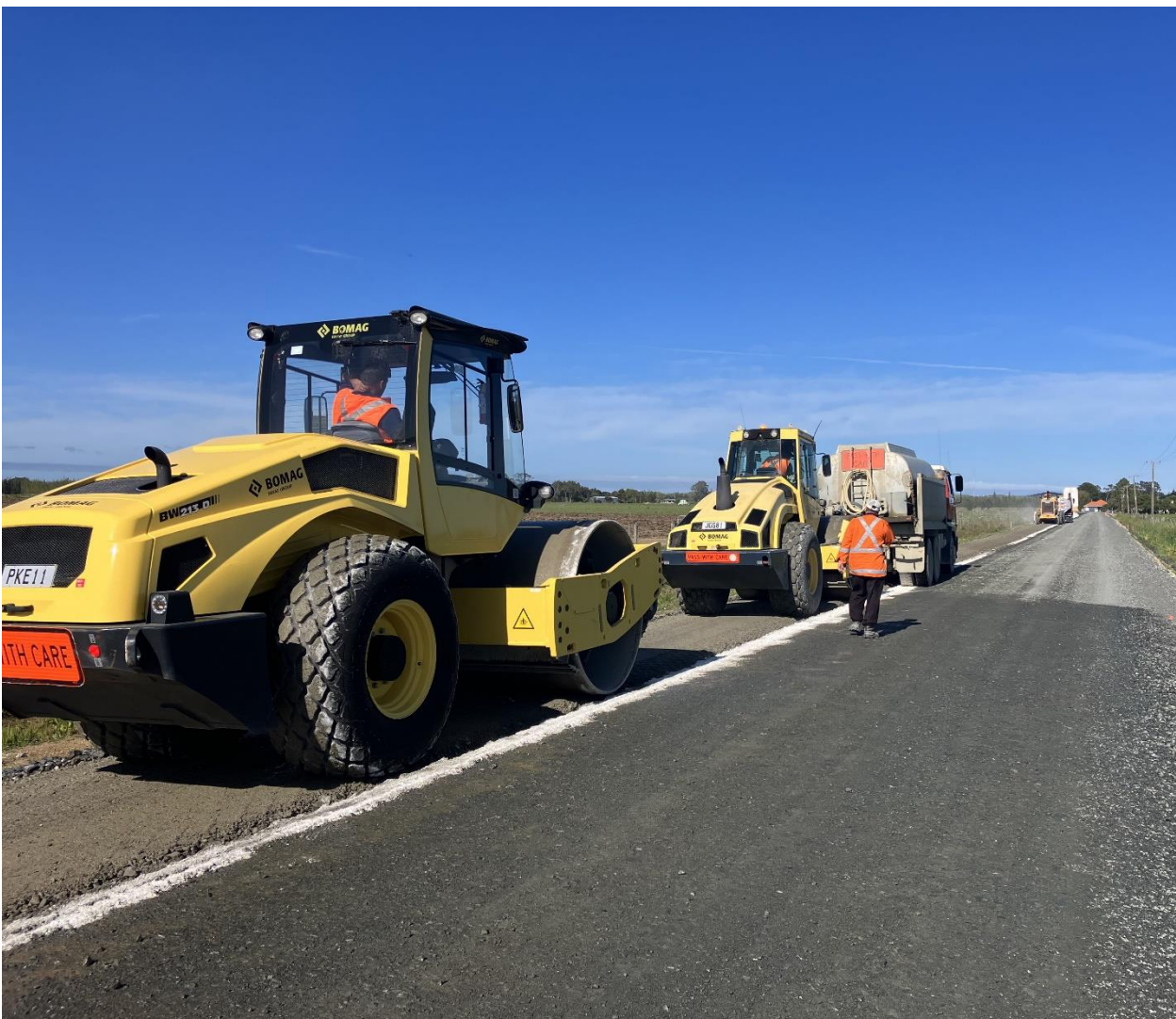
Stabilisation of the Gill Road Pavement Rehabilitation
