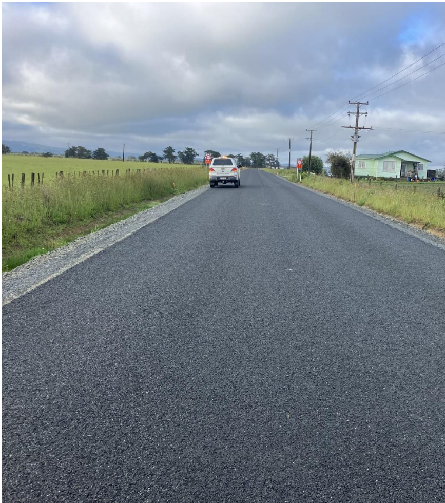
Gill Rd Pavement Rehabilitation Seal
