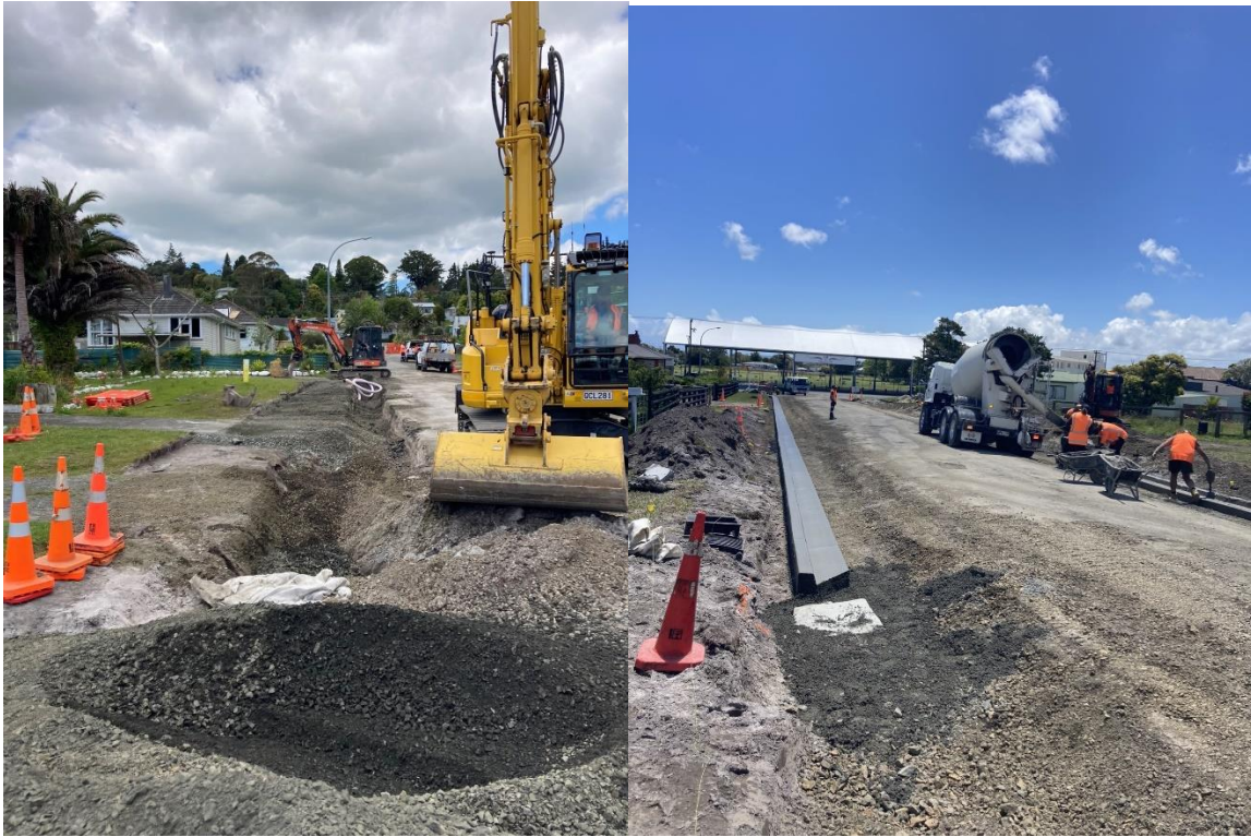
Sommerville Ave SW Upgrade Kerb and Channel and Footpath Preparation
