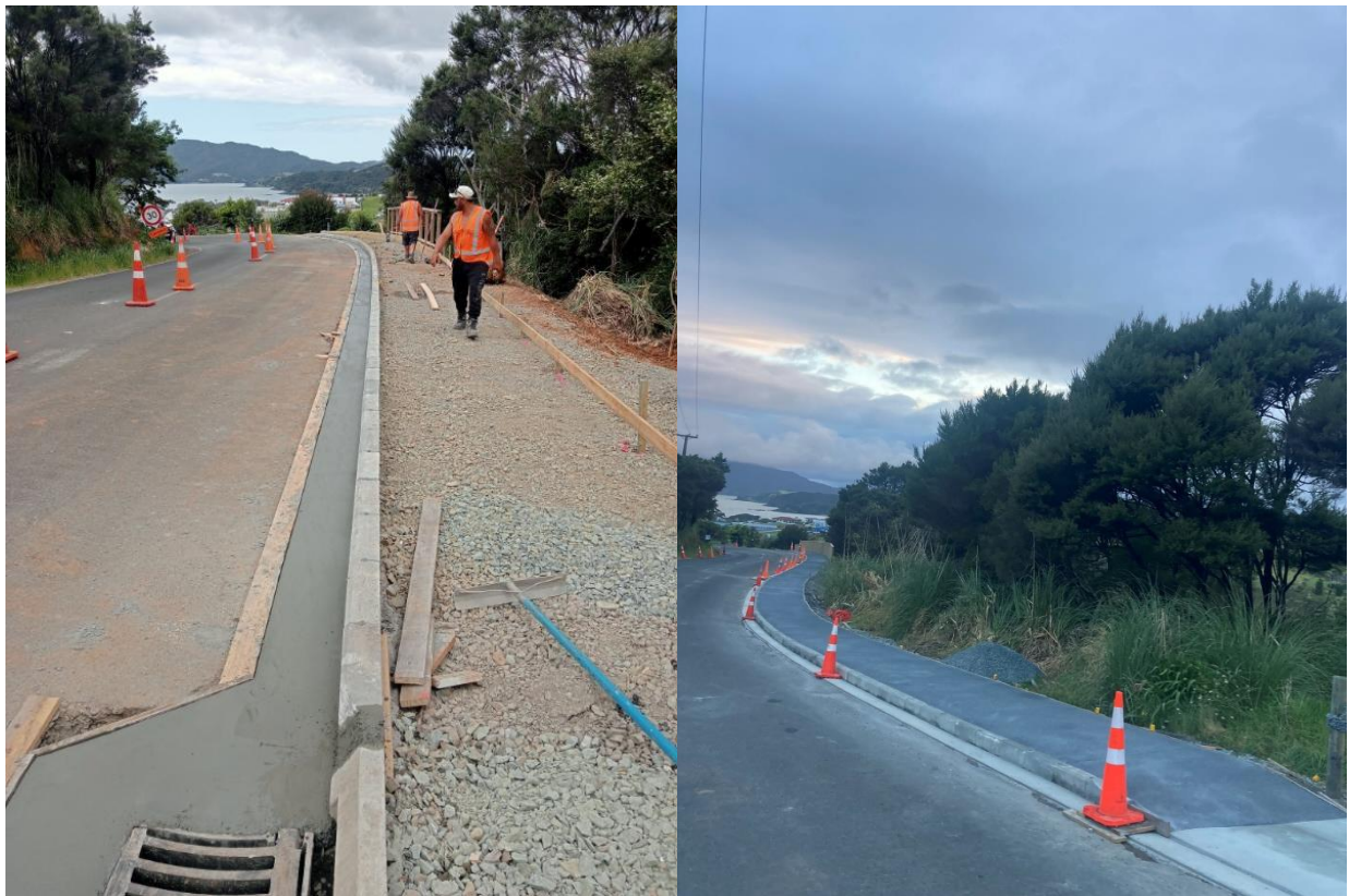
Cable Bay Block Road New Footpath
