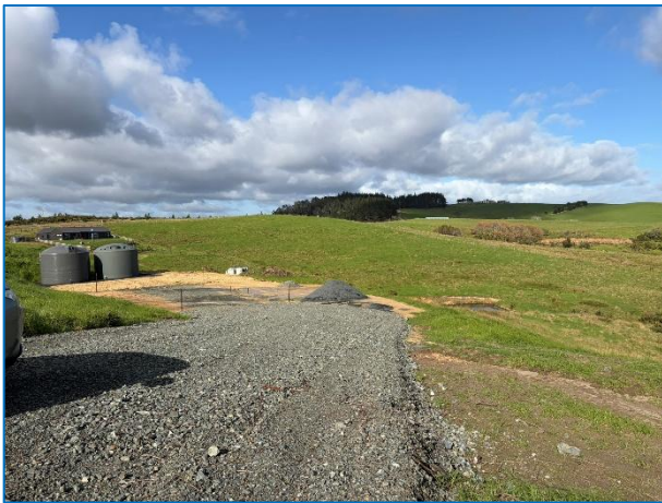
Photograph 1: Prepared driveway, building platform, water tanks and wastewater treatment system on Lot 1.
