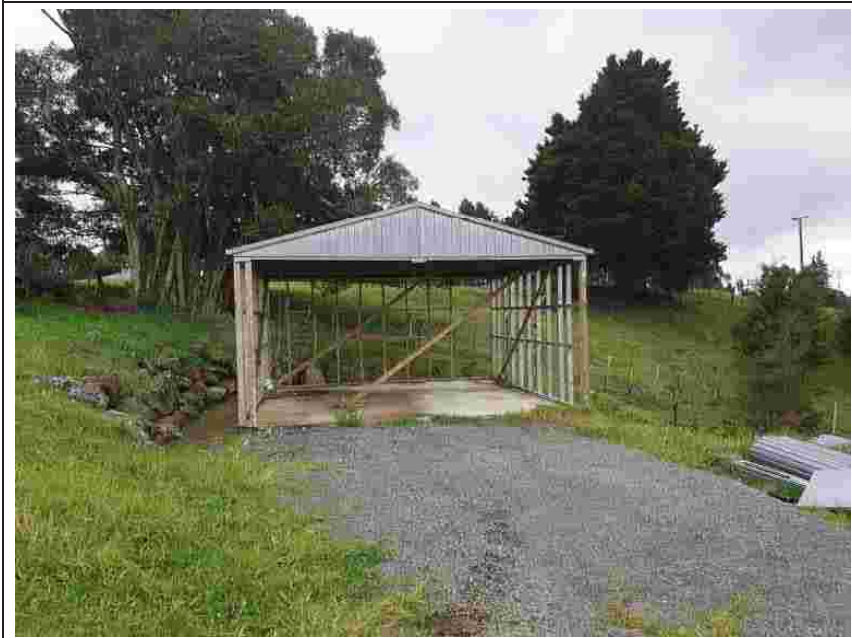
Photo 6: Low rock retaining wall upslope of half built garage. Gully feature visible behind and right of garage
