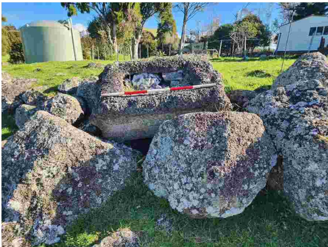
Figure 24: Underside of concrete chimney base strip footing and volcanic boulder core, looking southwest to the garage.
