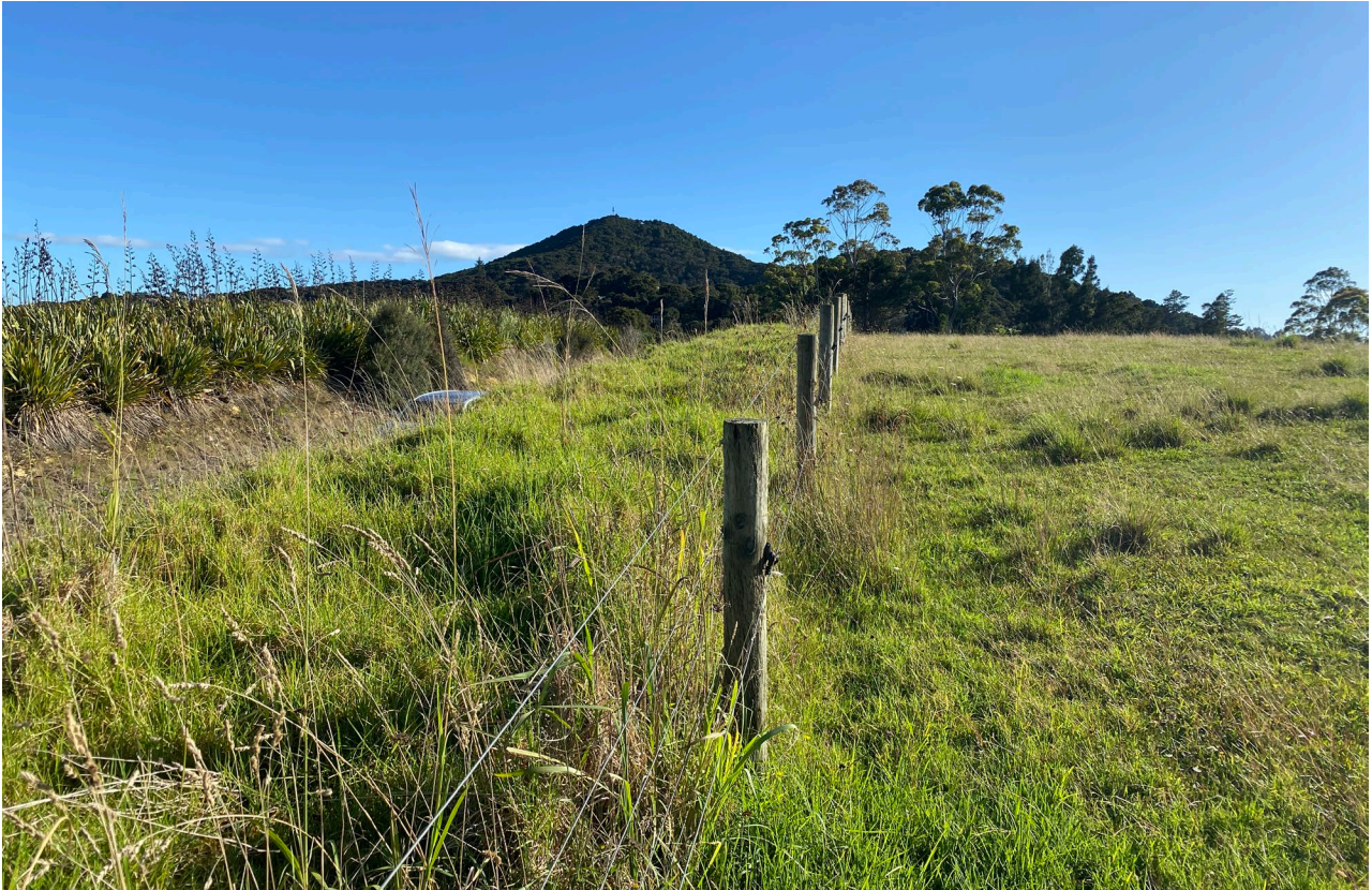
Photograph 5: View along part of Lane Road. The road has been cut through hillside obscuring the development from the road at certain locations.
