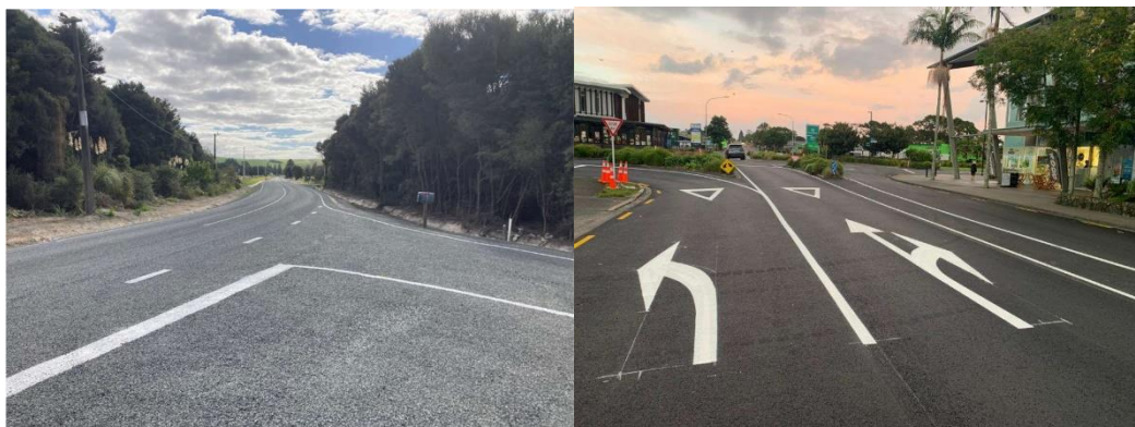
Left: Line marking on Parapara – Toatoa Road completed seal extension
