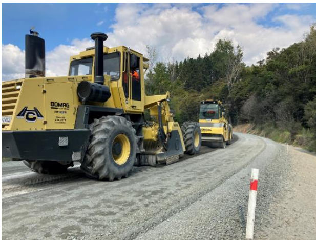
Figure 8: Kohukohu Rd Rehab Stabilisation
