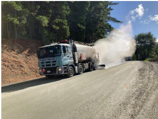
Figure 17: Kohukohu Rd Rehab Sealing
