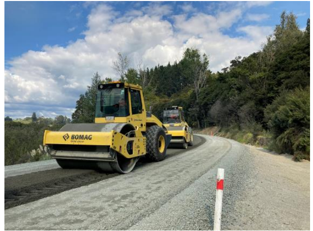
Figure 7: Kohukohu Rd Rehab Stabilisation
