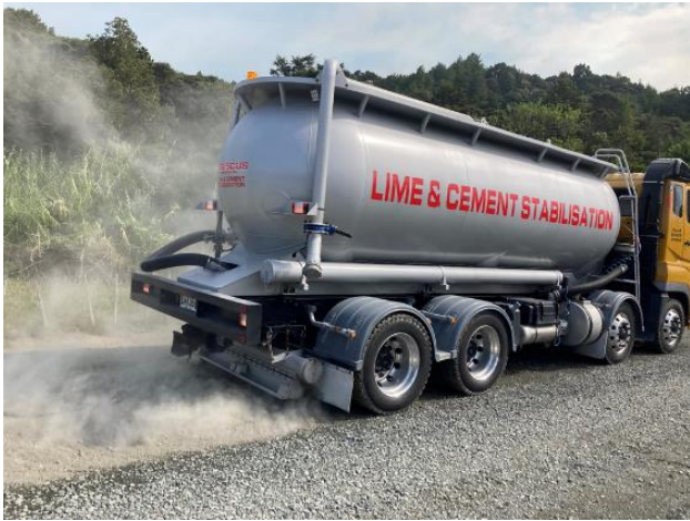
Figure 6: Kohukohu Rd Rehab Stabilisation
