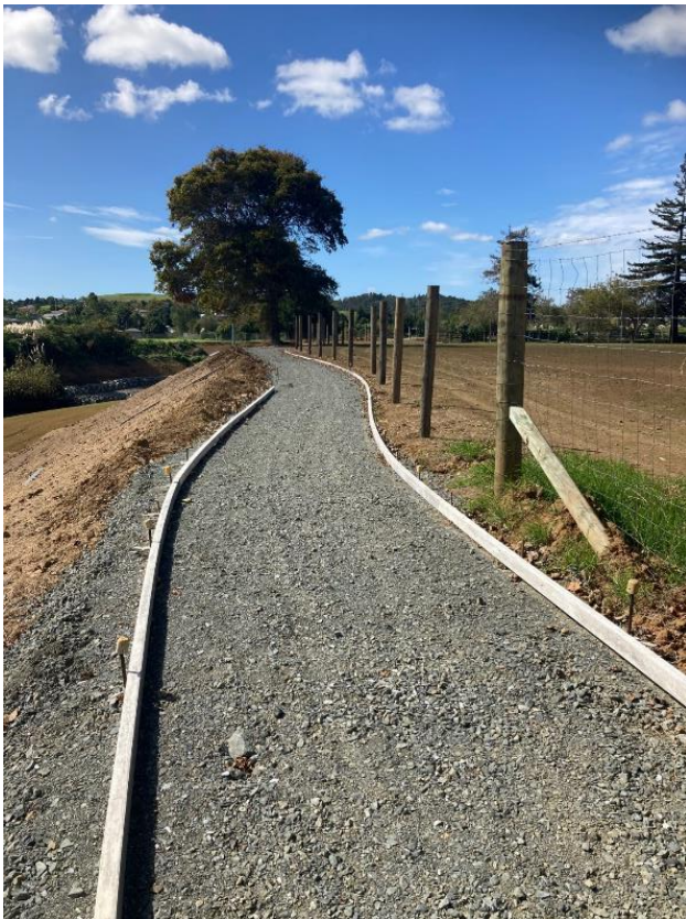
Figure 14: Te Ahu Footpath Construction
