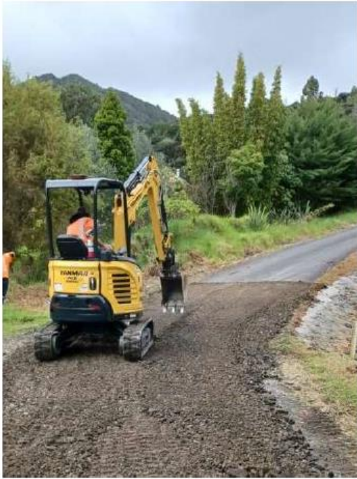
Waihuka Rd – Pavement Repairs
