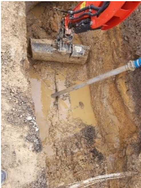
Omaunu Rd Kaeo AC sewer line beak repair.
