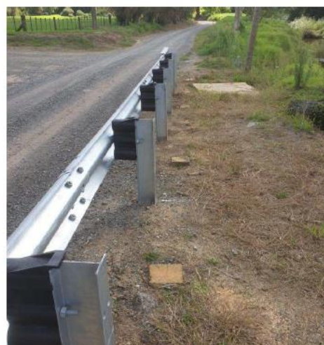
Tirohanga Rd – Guardrail Installation
