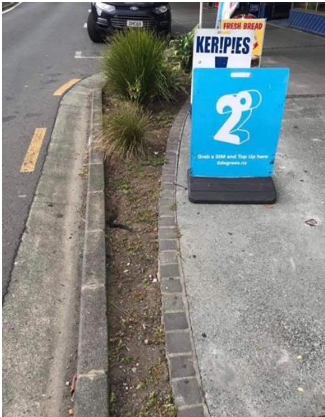
Outside Central Dairy BEFORE ....
