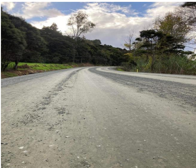
Figure 4: Kohukohu Rd Rehab Seal Prep
