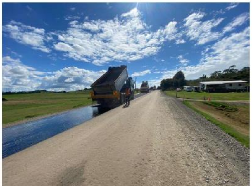
Chip sealing day – Waimatenui Rd
