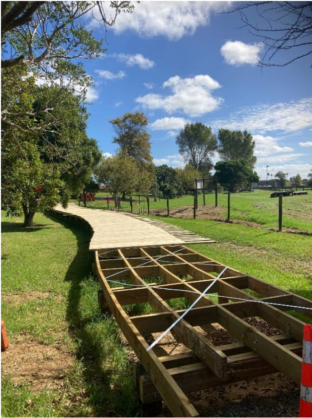
Figure 16: Te Ahu Footpath / Board Walk Construction
