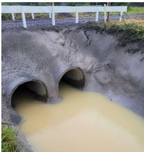
Wahamiti Lane – Headwall Shotcrete
