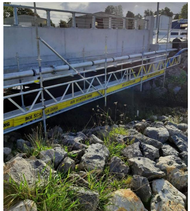
Waipapa Bridge Crossing This project is part of a major road work project with a requirement to realign water mains and divert all connections
