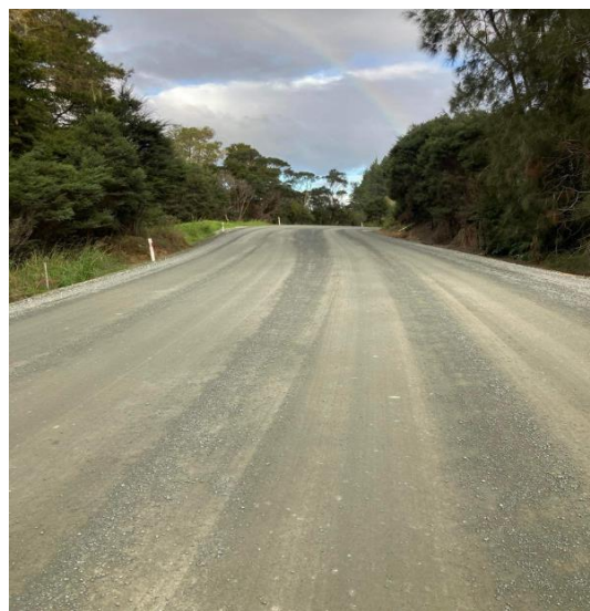
Figure 5: Kohukohu Rd Rehab Seal Prep
