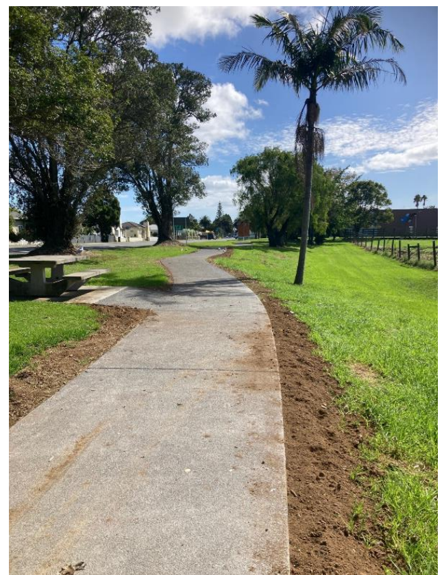
Figure 15: Te Ahu Footpath Construction
