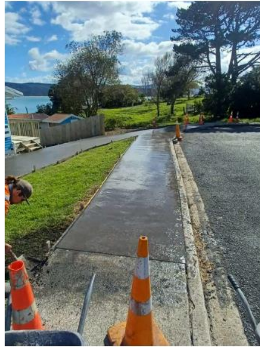
Fairlie Cres – Footpath Replacement
