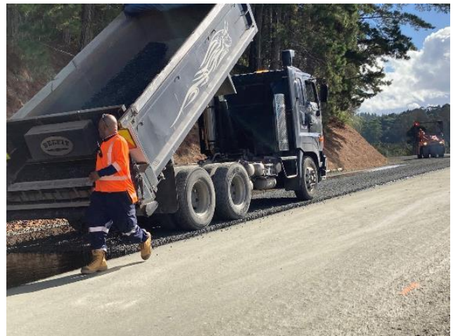
Figure 18: Kohukohu Rd Rehab Sealing
