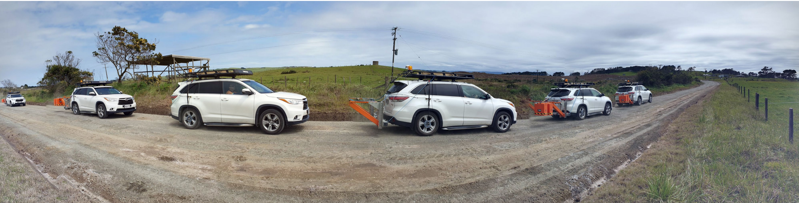
Photo: Ground Penetrated Radar (GPR) use to measure existing pavement depths
