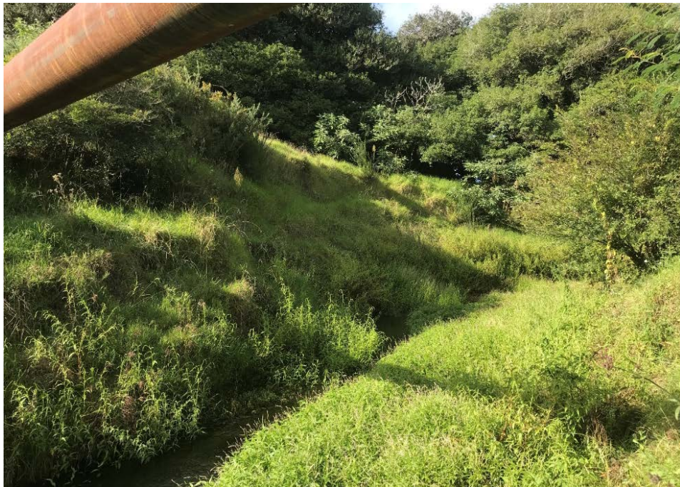
Photograph 6. Waihoe Channel. Looking upstream.
