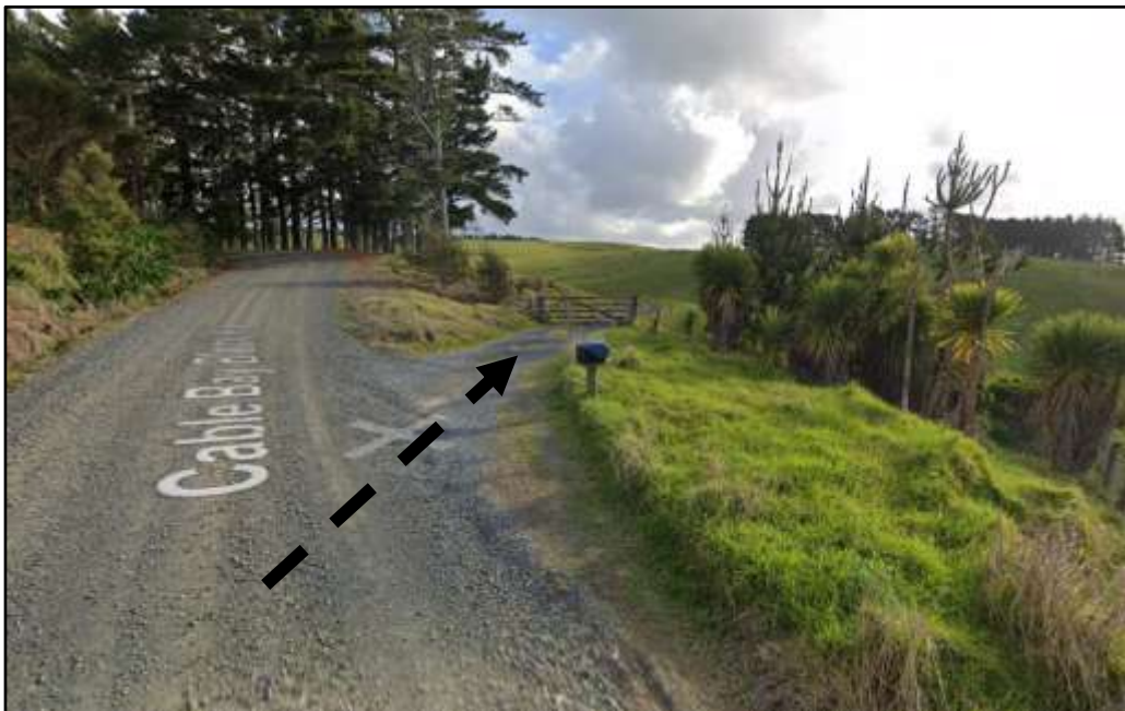
Figure 5: Vehicle Crossing on Cable Bay Block Road (Source: Google Streetview).
