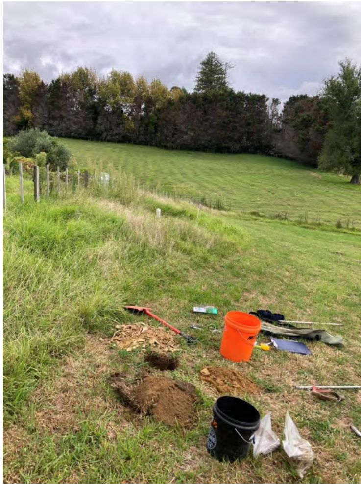
Figure 1: Subsoil Investigation Near the Existing Trench
