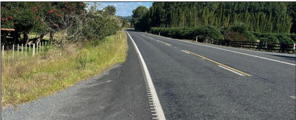
Figure 2: View to the North/West
