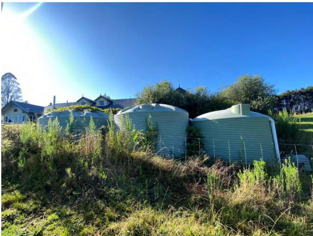
Figure 2: Existing Water Tanks
