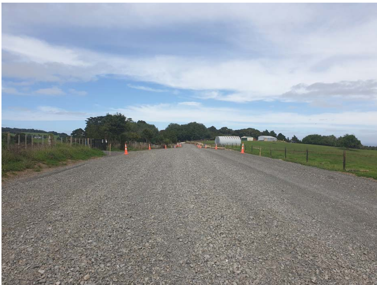
Ruapekapeka Road Stage 1 pavement construction
