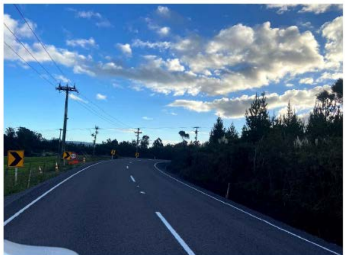
Pungaere Rd – Sealing and after photo
