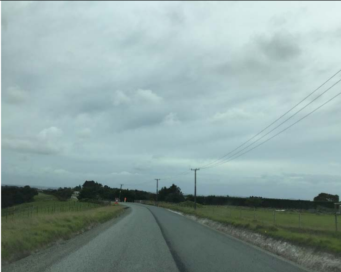
Church Road/ Seal Extension – Fresh Seal
