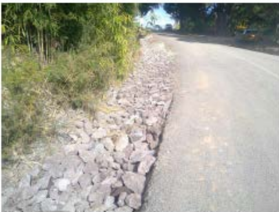
Ngawha Springs Rd – Scouring repairs
