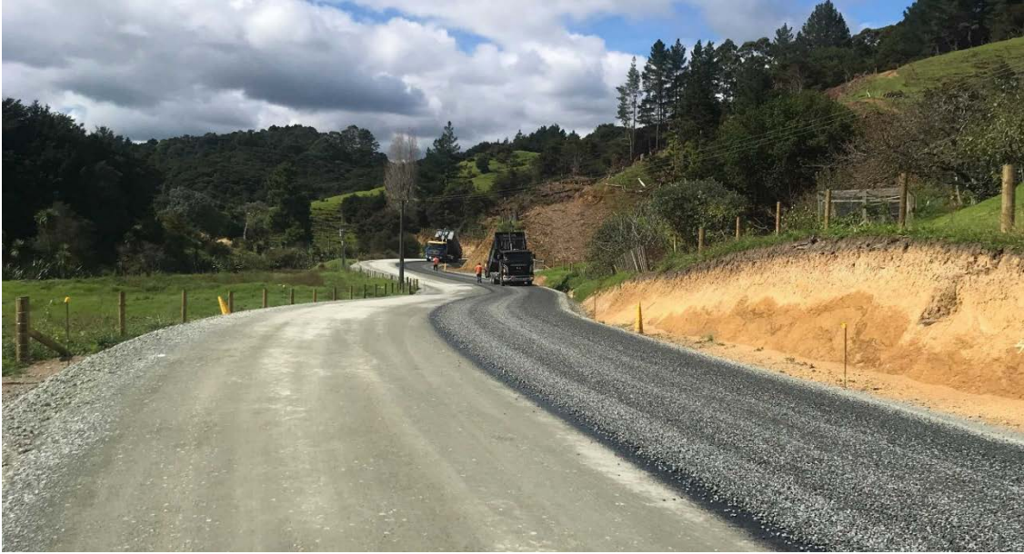
Sealing at Peria on Section 4
