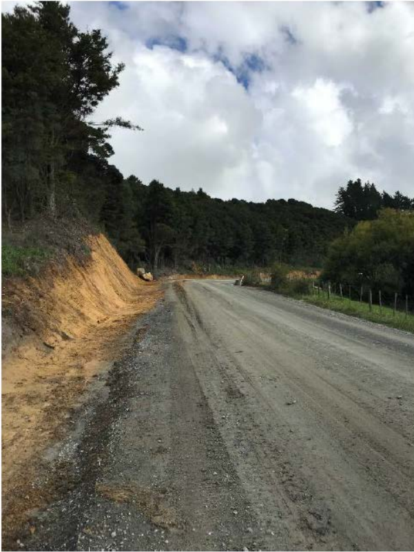
Figure 4: Section Five Clearing
