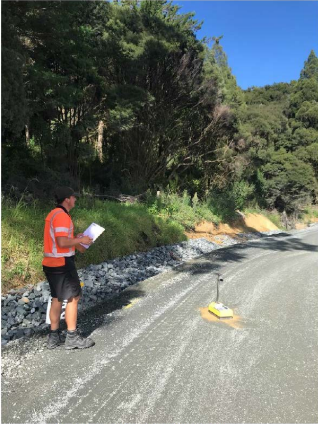
Figure 21: Section Four Nuclear Density Testing
