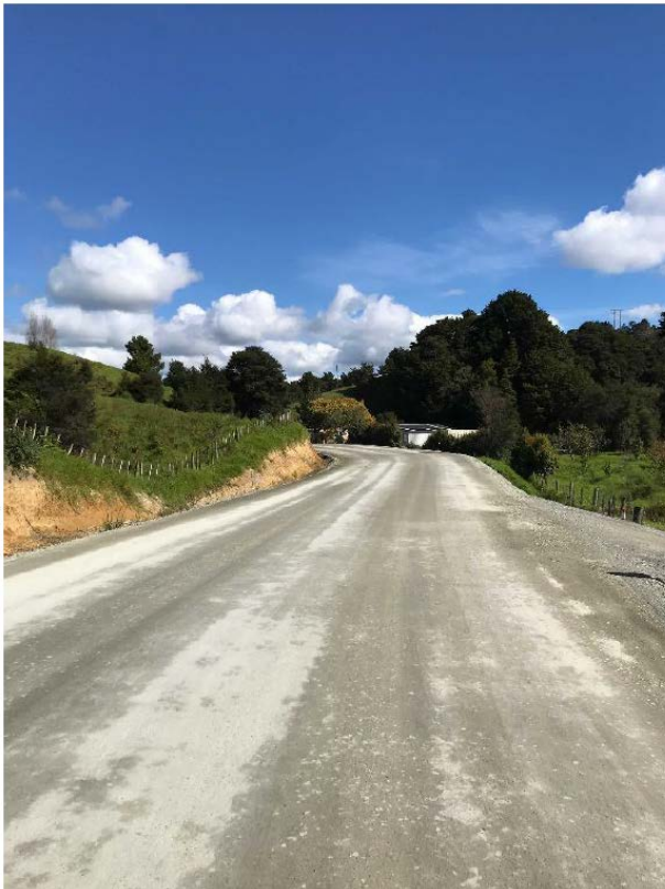
Figure 28: Section Four Ready for seal
