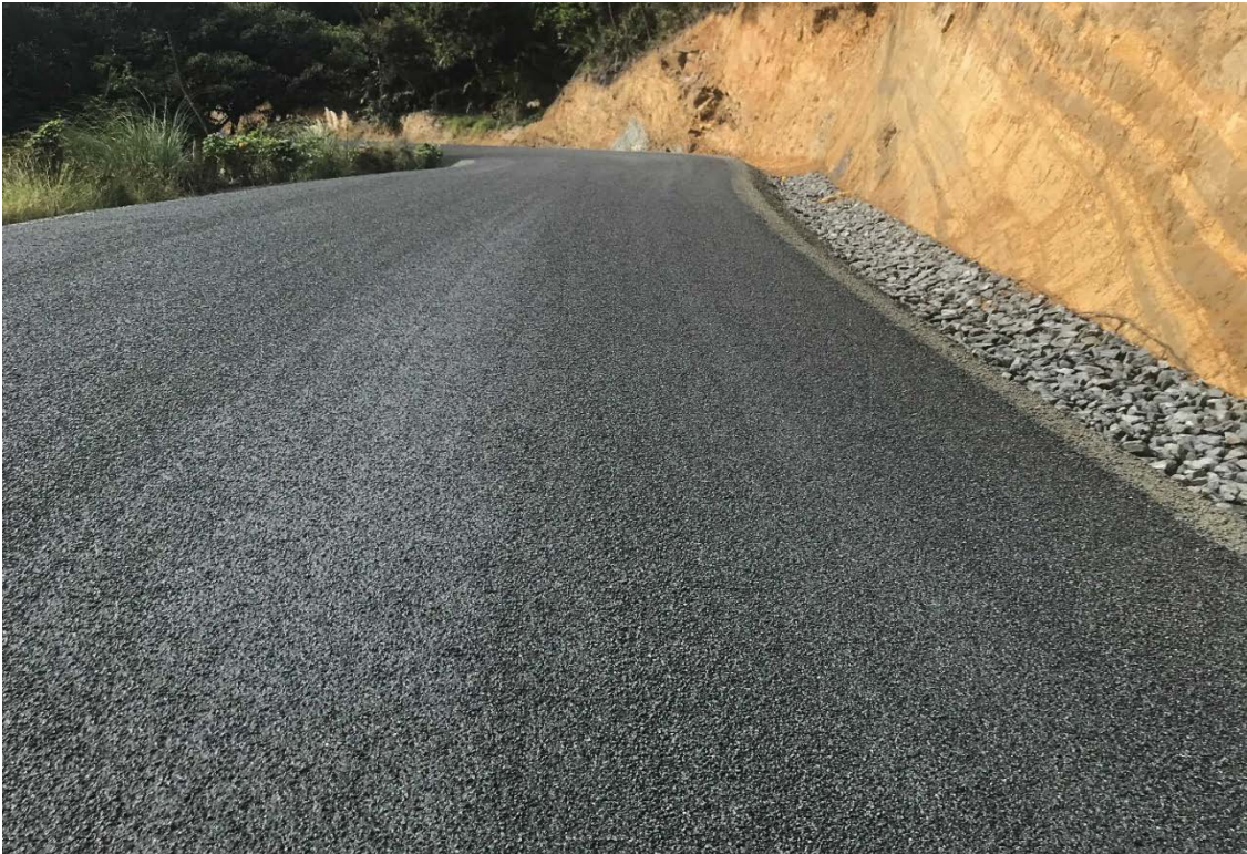
Final seal at Peria on Section 4
