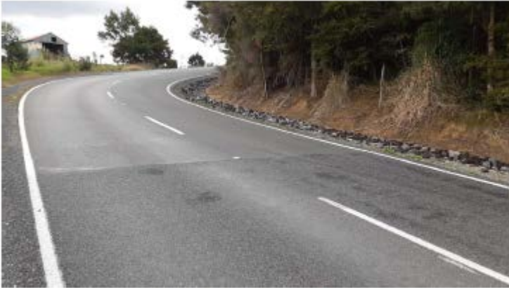
Callaghans Rd (Maromaku-Towai) – Scouring repairs
