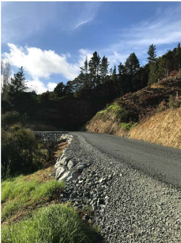
Figure 20: Section Four Seal Prep
