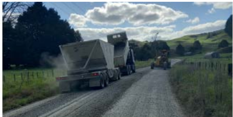
Orakau Rd – Maintenance Metalling
