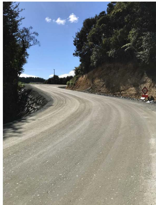
Figure 29: Section Four Ready for seal
