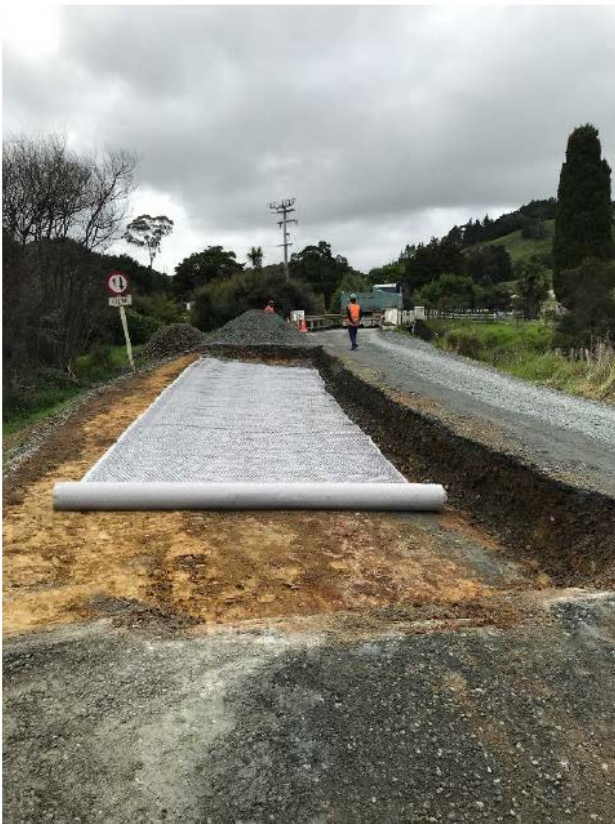
Figure 6: Section Five Bridge Undercut
