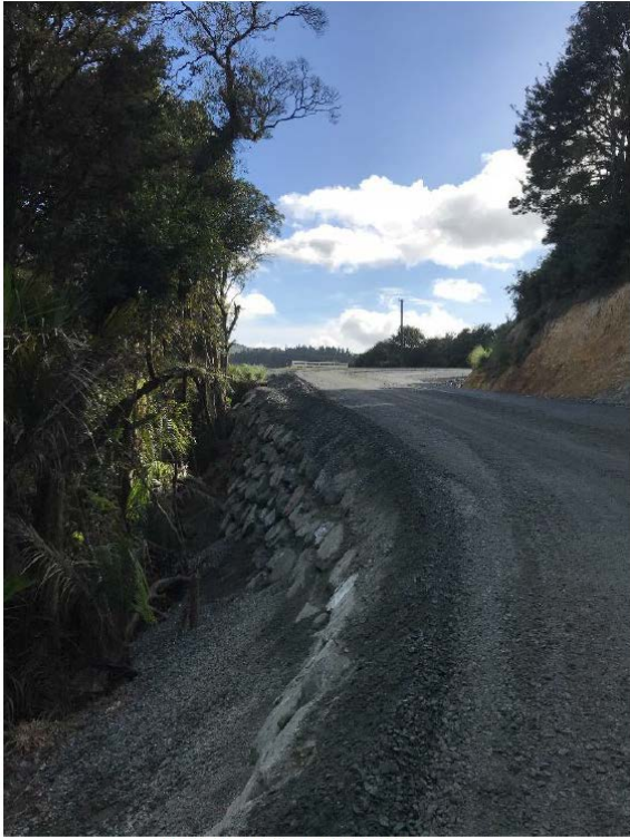
Figure 14: Section Four Seal Prep
