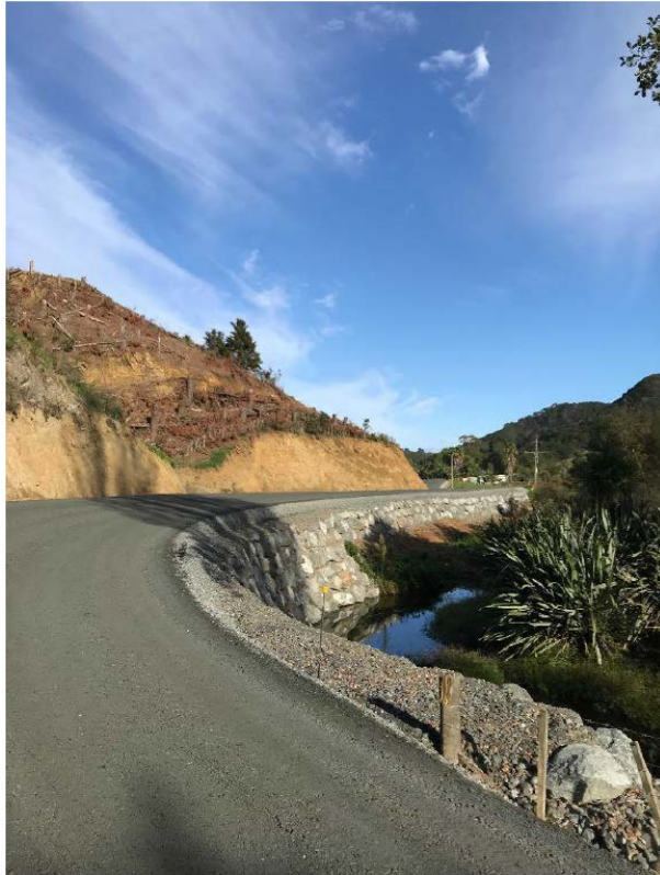
Figure 18: Section Four Seal Prep
