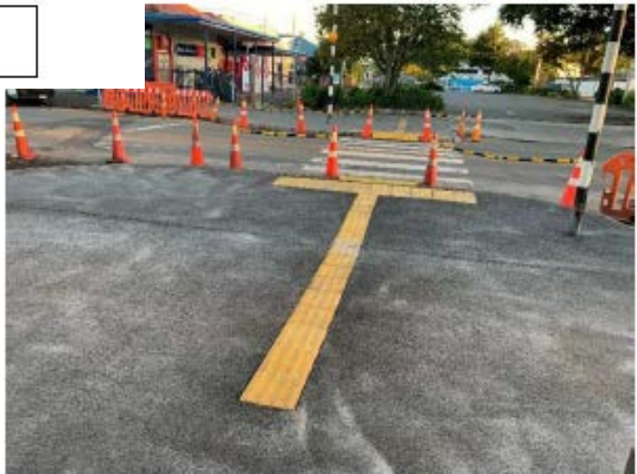
Hobson Ave – Brand New Pedestrian Crossing in progress
