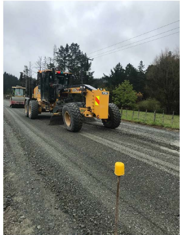
Figure 33: Section Five Pavement overlay
