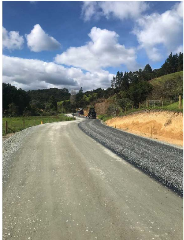
Figure 31: Section Four Seal in progress
