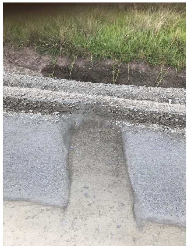
Figure 4: Great compaction all the way to edge of shoulder
