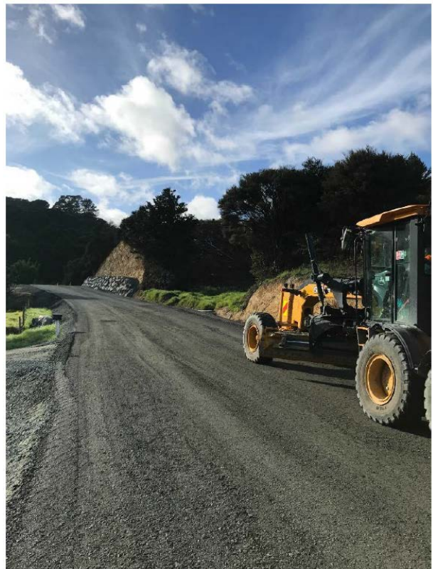
Figure 17: Section Four Seal Prep
