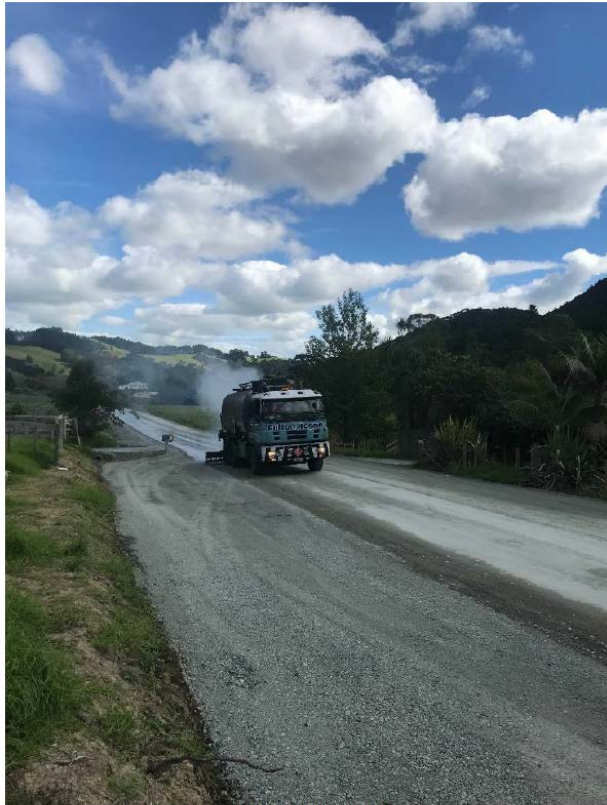
Figure 30: Section Four Seal in progress
