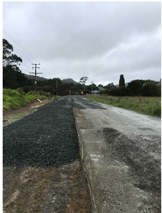
Figure 7: Section Five Pavement undercut
