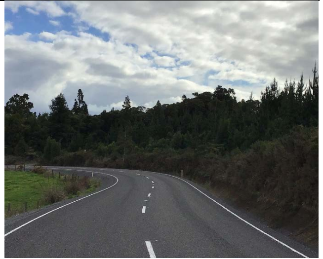
Pungaere Road/ Seal Extension – complete
