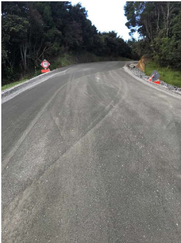
Figure 23: Section Four Seal Prep
