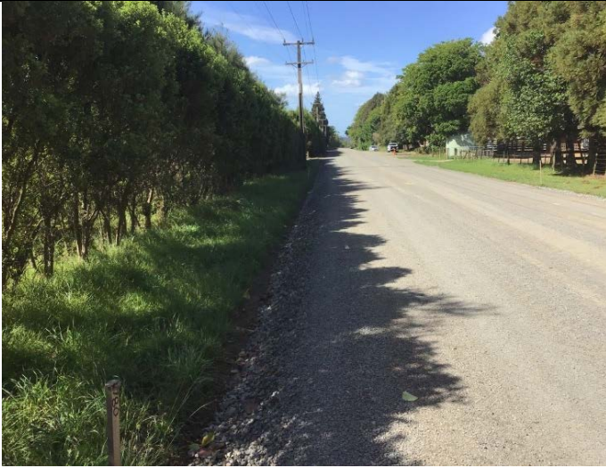
Koropewa Road/ Seal Extension – Pavement ready for sealing
