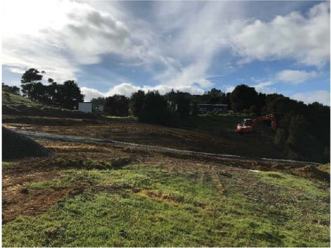
Figure 15: Section Four Tip Site Tidy Up
