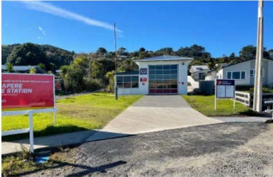
Omapere Fire Station – Asphalt tie in
