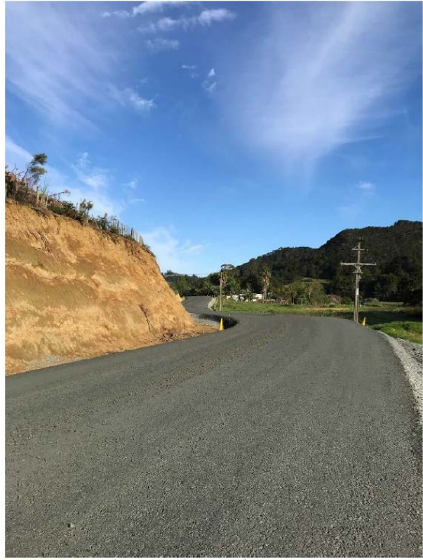
Figure 19: Section Four Seal Prep
