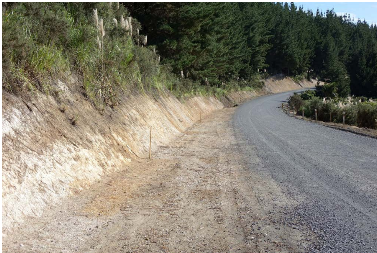
Ngapipito Road clearing/earthworks and survey/set-out completed on sections 1 & 2
