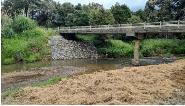
7/21/215 SP3 – Scour Protection Works at Pipiwai Road Bridge W08
