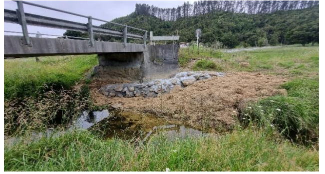
7/21/215 SP3 – Scour Protection Works at Matawaia-Maromaku Road Bridge W22
