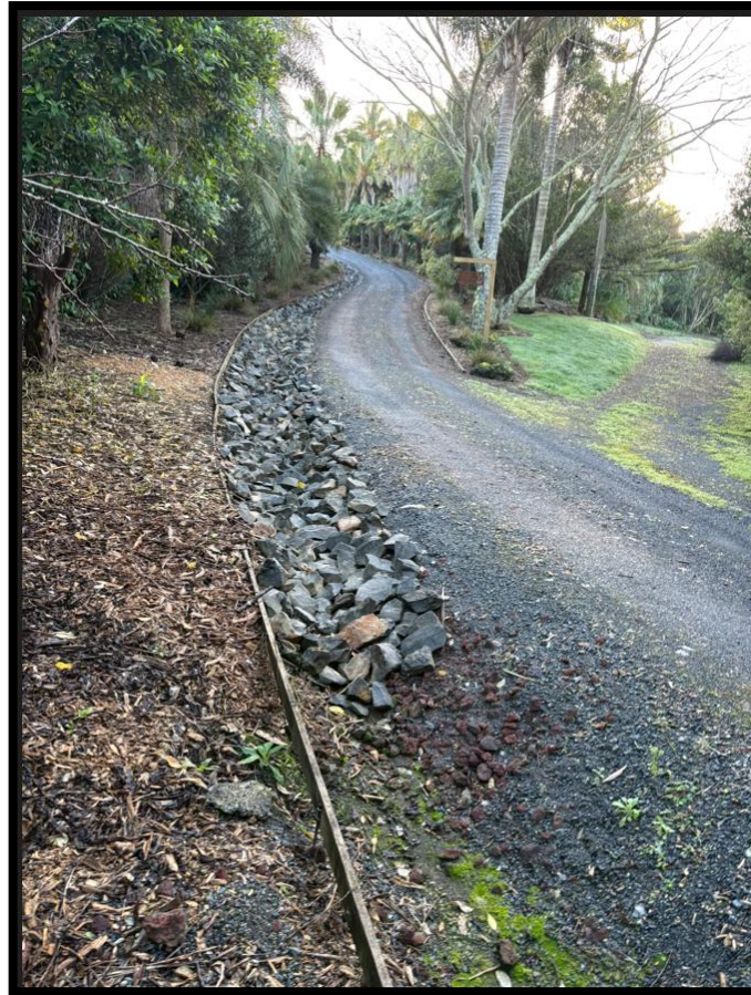
Figure 6 – Existing riprap rock lined channel adjacent to driveway with neighbouring driveway to the right
