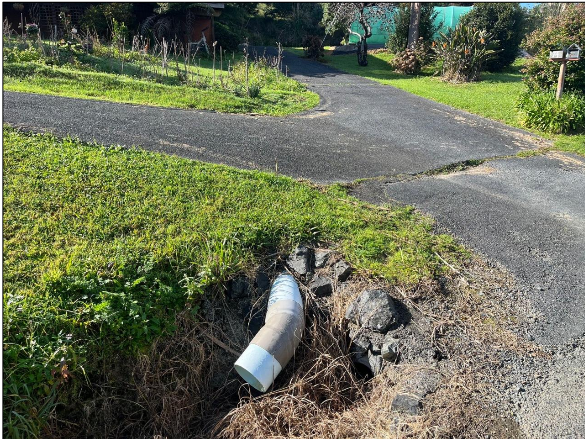
Figure 6: 07.07.2025 Site Photo – View of sump (background, at top of vehicle crossing) and existing outlet to roadside drain (foreground).
