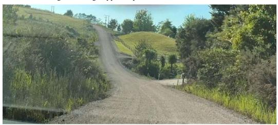
**Photo 5**. Looking west along Wakelin Road towards the SH10 intersection and the start of the seal and showing the poor advance warning of the presence of the intersection. The speed limit transition is for 60 km/hr on Wakelin Road
