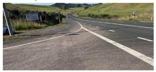
**Photo 7.** Looking north along SH10 from Wakelin Road. It is proposed to address the minor visibility restriction in this direction by replacing the sign shown in Photo 8 with a WJ5L "intersection ahead" permanent warning sign.
