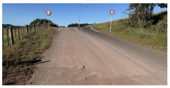
**Photo 6.** Looking south along SH10 from Wakelin Road. Note the passing lane and taper. Excellent visibility
