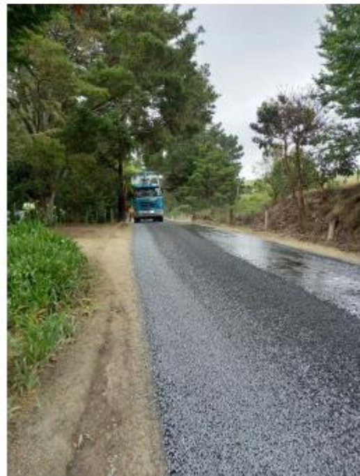
Umarewa School Rd – Dust Sealing site
