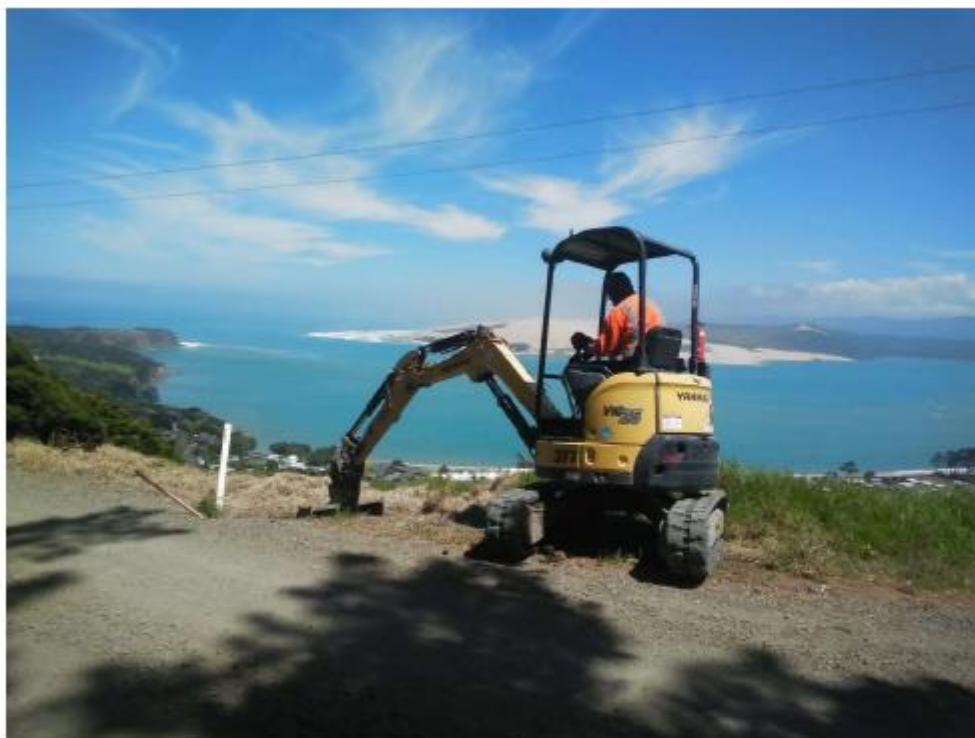
Routine Culvert Clearing – Not a bad view – Newton Rd
