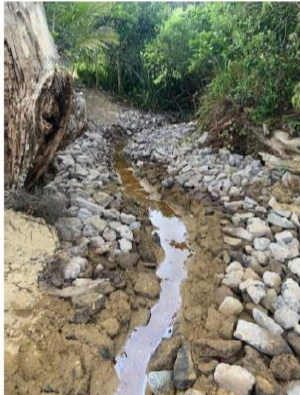
Te Uenga Bay – Culvert outlet to Beach foreshore
