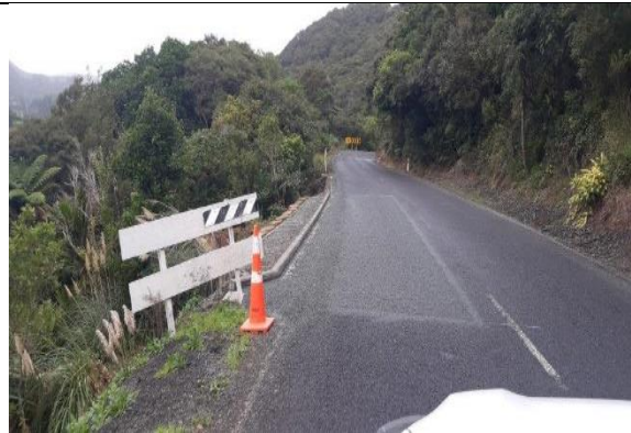
Kaitaia Awaroa Road – Completed timber pole retaining wall
