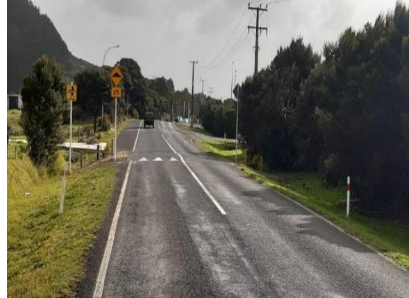
Ahipara Road - First traffic calming raised platform before entrance into Ahipara township
