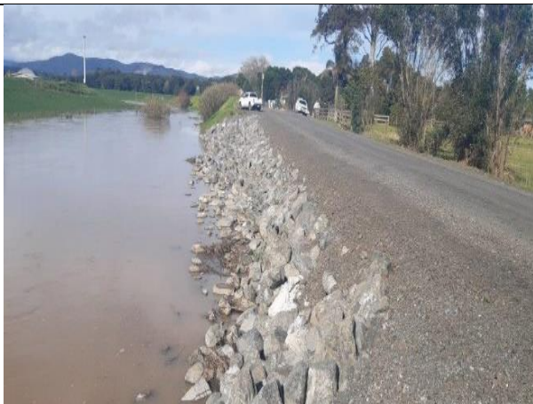
Gill Road – Completed profiled rock wall retaining structure
