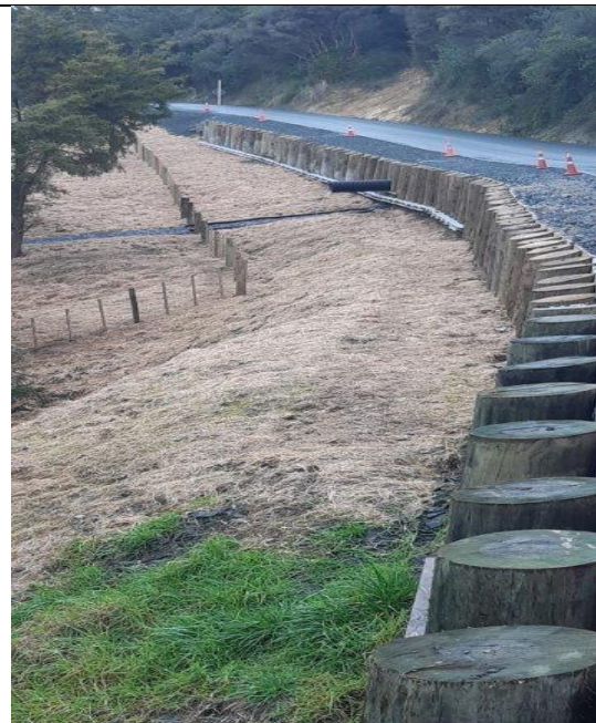
Fairburn Road – Completed anchored timber pole retaining wall
