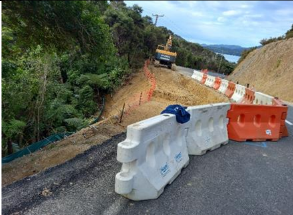
Manawaora Slip Repair – Cut bench & setting out of production soil nails
