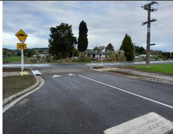
Moerewa LATM - Raised safety platform and kerb build out at Nisbet/Otiria intersection (permanent line marking yet to be completed)
