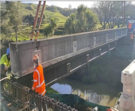
Churtons Road bridge replacement – Ongoing beam installation
