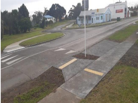
Takahe Rd, Ahipara Raised - traffic calming platform, footpath connection & driveway upgrade
