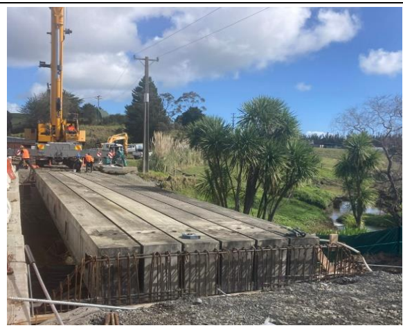
Churtons Road bridge replacement – Ongoing beam installation
