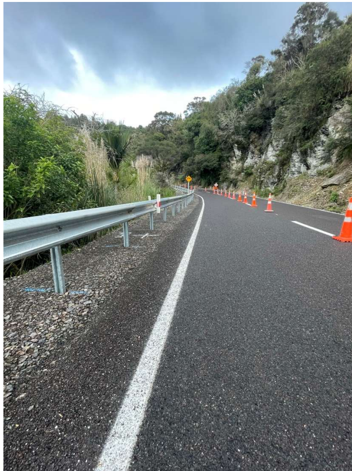
Mangamuka Road Guardrail Installation
