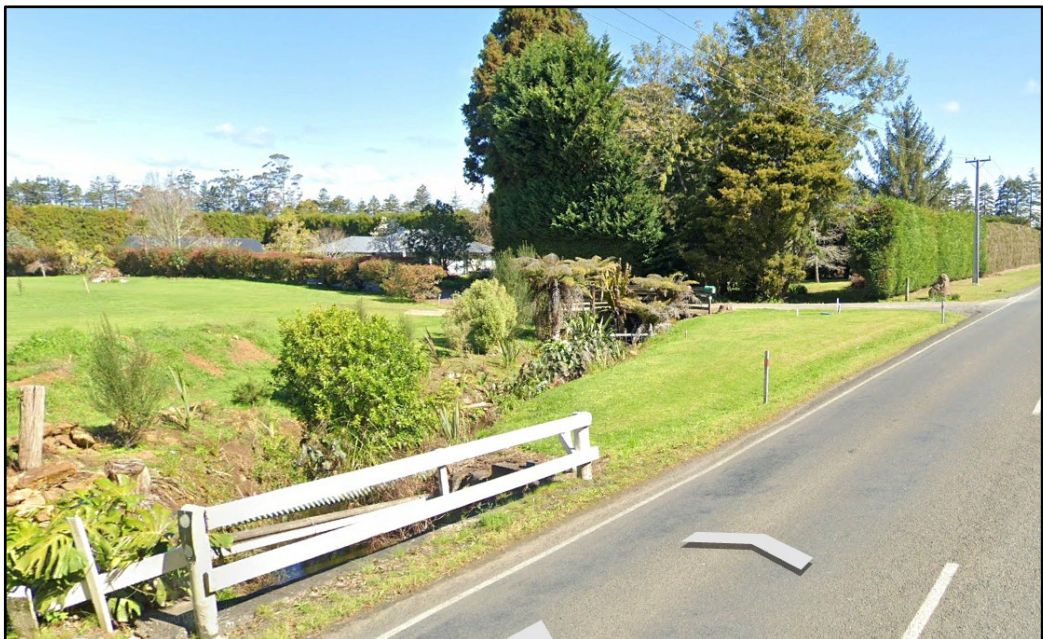
Photograph 1: Stream running under Kerikeri Inlet Road and through subject land
