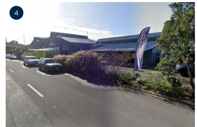
4 Marine industrial / commercial A marine commercial hub is located on the western edge of the marina.
