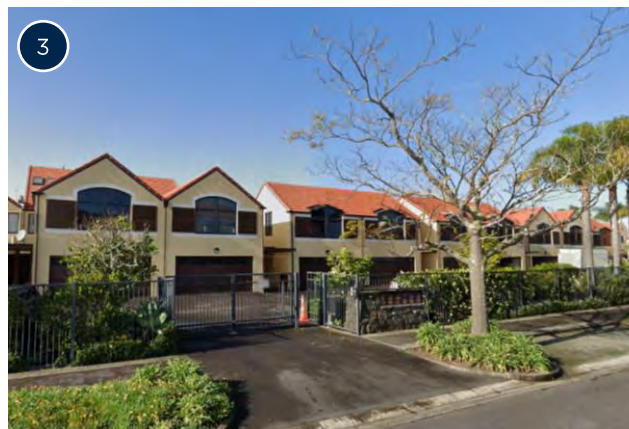
3 Residential / accommodation (low rise) Various examples of terraced style housing alongside the more substantial apartments.
