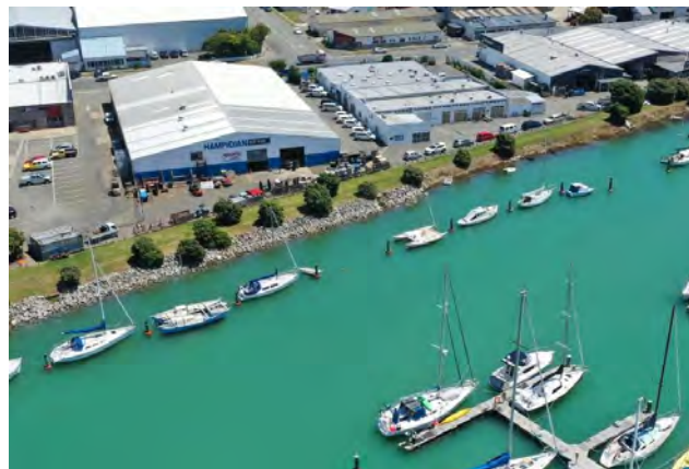
Commercial on Port Nelson land There are various larger commercial premises located immediately opposite Nelson Marina on Port Nelson land.
