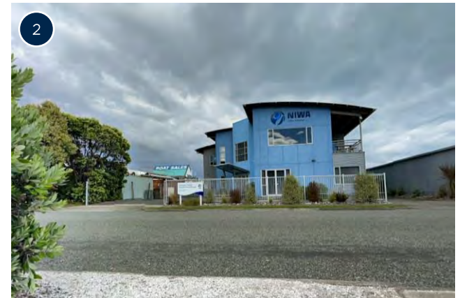
Commercial Some examples of commercial properties located alongside the marina. These are marine related.
