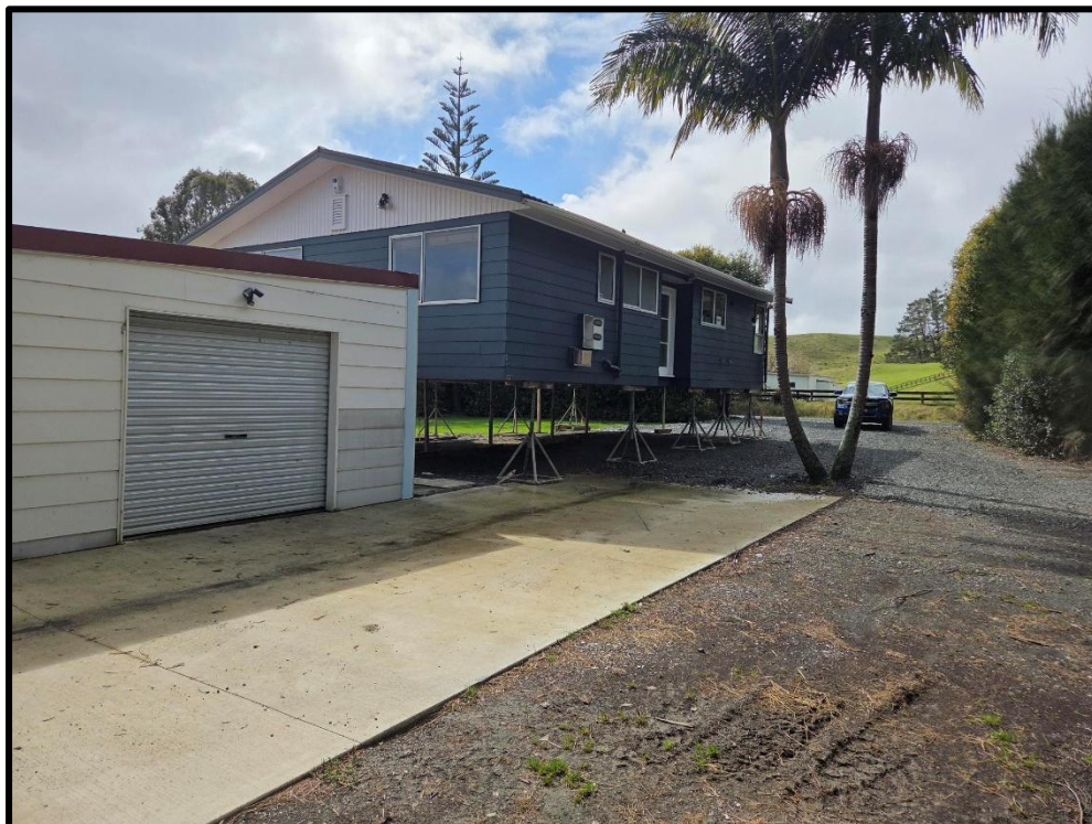
Figure 6: Existing garage and relocated dwelling, looking towards entrance from Godinovich Road.
