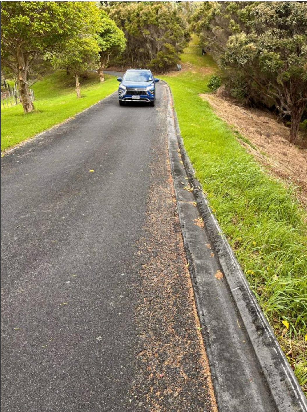
Lot 3 ROW localised seal damage (perished) and minor settlement (rotation of kerb and channel)
