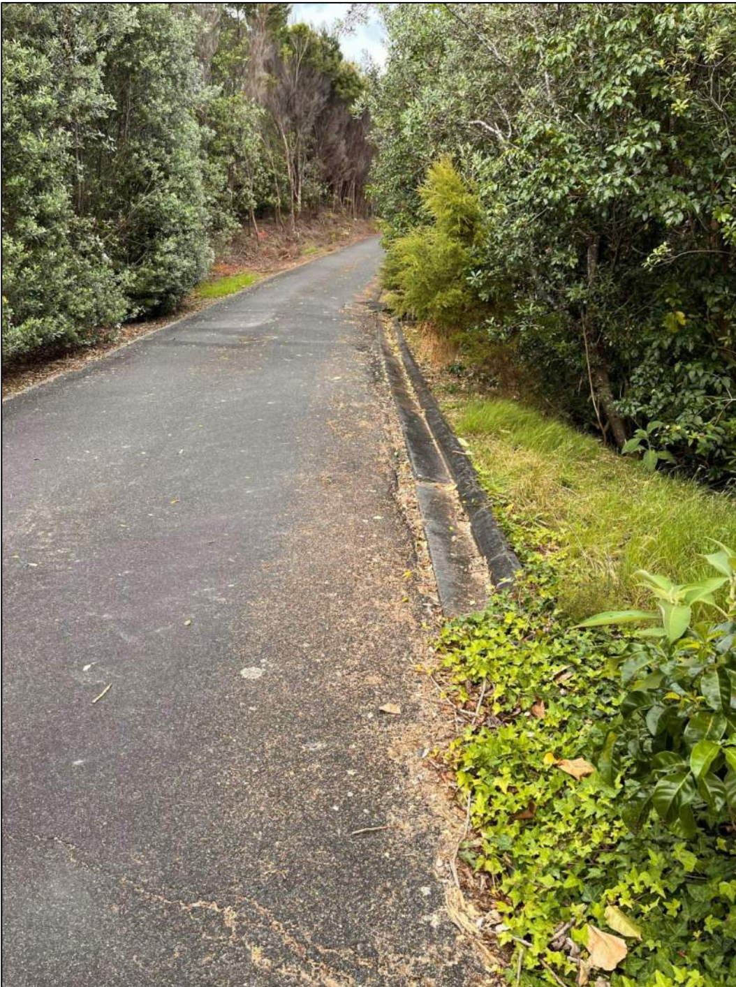
Lot 3 ROW localised seal damage and more pronounced settlement (rotation of kerb and channel)
