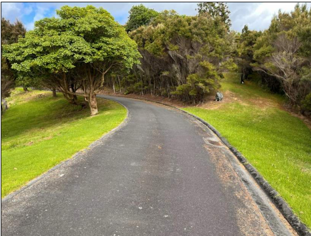
Lot 3 ROW typical 3.9m width, seal coated, nib and kerb and channel with cesspit and culvert drainage
