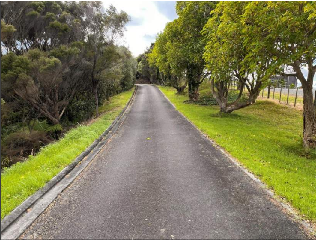
Lot 3 ROW typical 3.9m width, seal coated, nib and kerb and channel
