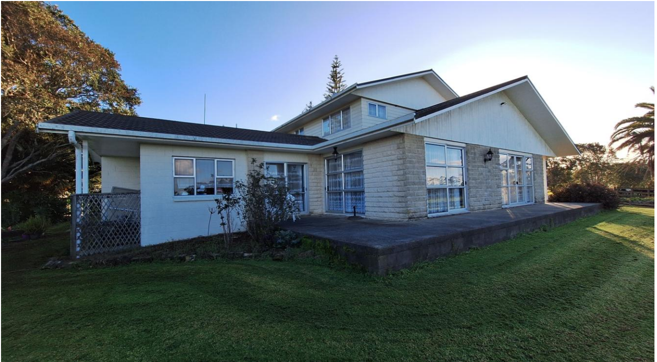
Existing dwelling and patio from eastern garden.
