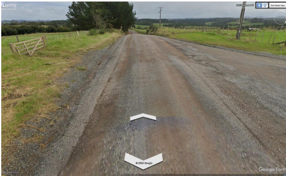
Figure 3: Site distance to the South (source: google street view)
