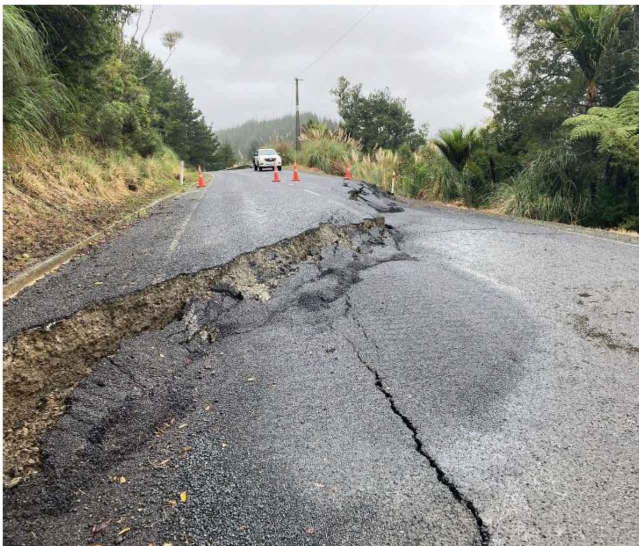
Underslip at West Coast Rd (near to Motuti Road), the main route between Kohukohu and Panguru.
