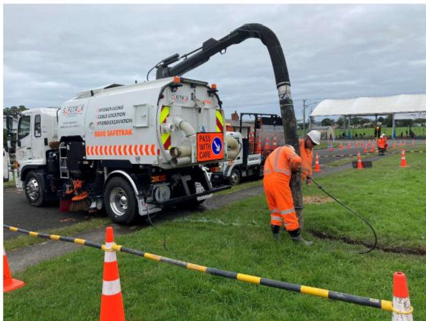
Service locations completed for Sommersville Ave Stormwater Replacement and Pavement Rehab.
