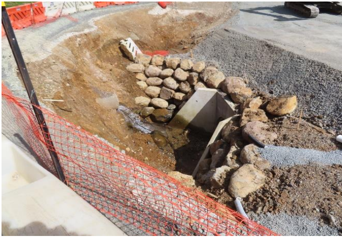
Figure 4) 2100 culvert inlet and outlet wingwalls
