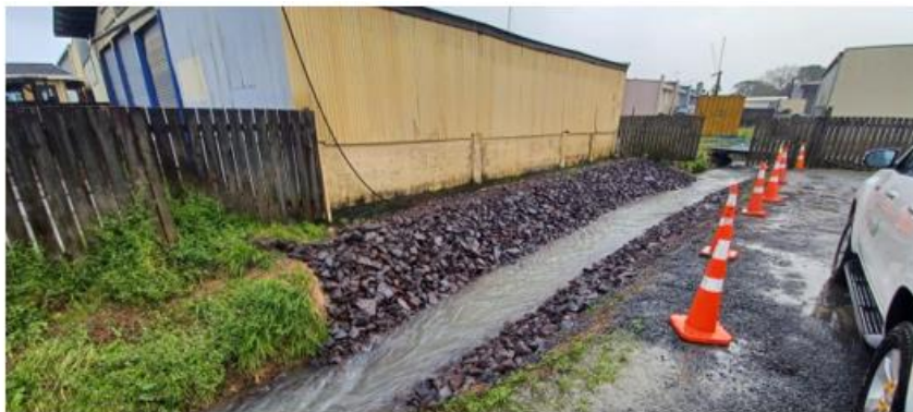
Mill Road, Kerikeri Stormwater Stabilisation
