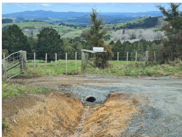
Figure 2) Driveway culvert crossing
