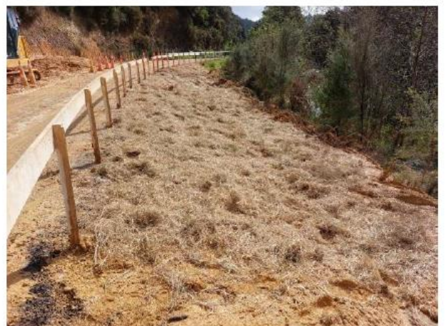
Step 5 – tidy up road and clear away remaining material with ditch witch. Stabilise exposed clay areas.
