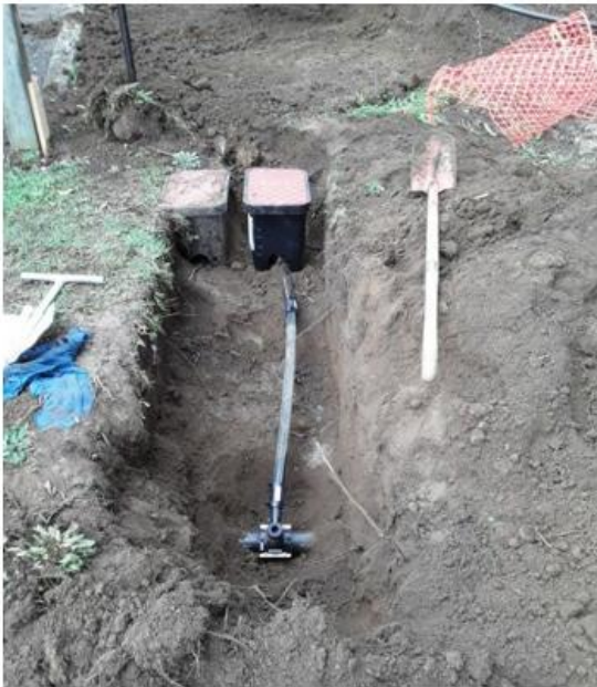
New LPS Sewer Connection – Kerikeri
