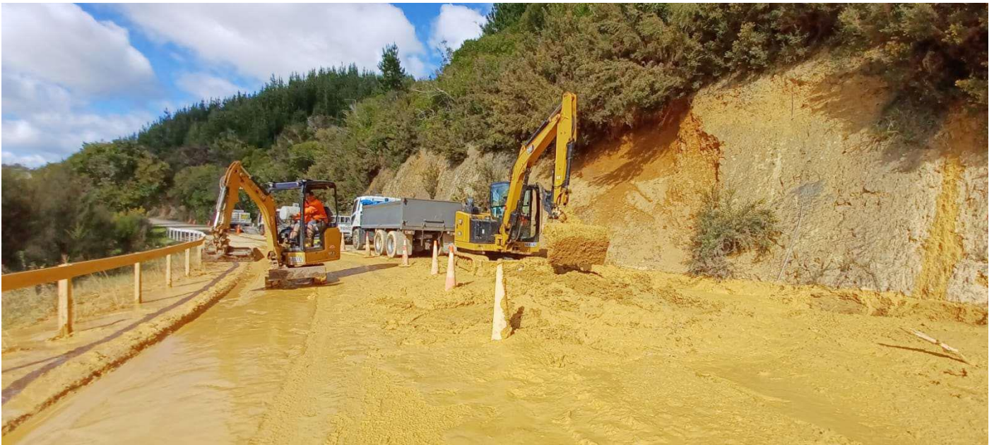
Step 5 – tidy up road and clear away remaining material with ditch witch. Stabilise exposed clay areas.
