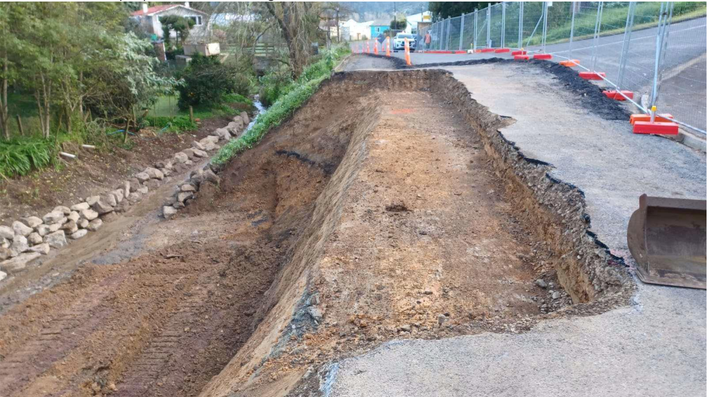
3. Commercial St Slip repair and stream realignment – FNDC/NTA
