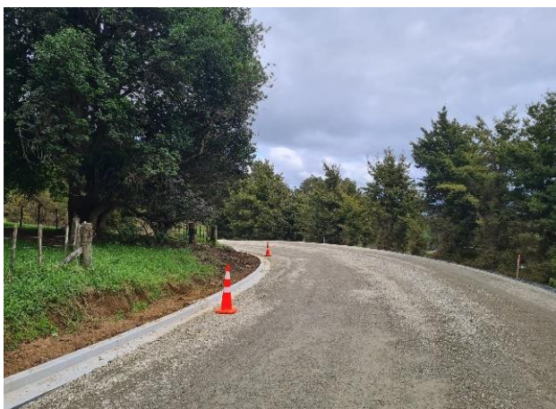
Figure 2) Kerb and channel
