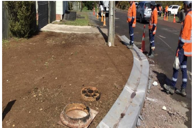
Ngawha Springs Road Rehabilitation Drainage works started
