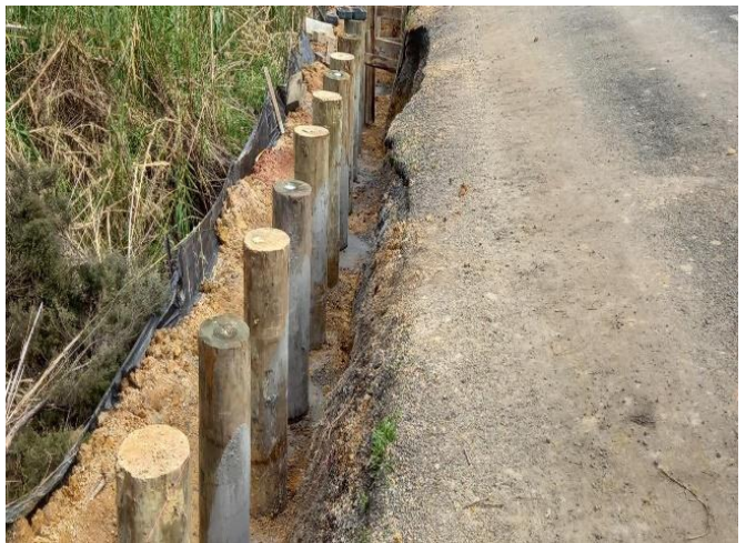
Aucks Road Slip Repair, Russell
