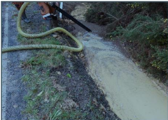
Step 5 – tidy up road and clear away remaining material with ditch witch. Stabilise exposed clay areas.
