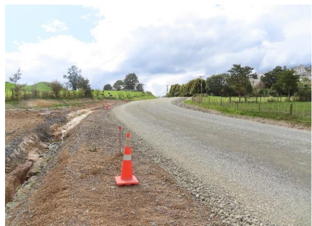
Figure 3) Basecourse ready for compliance testing
