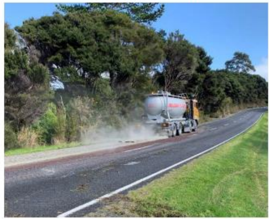
rua - Spread Cement
