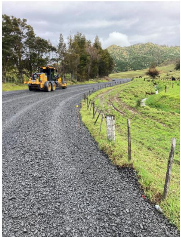
Figure 10: Pawarenga Rd Rehab Pavement Overlay
