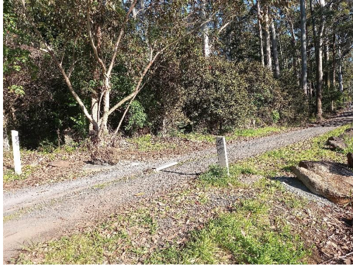
Rocks concreted into position at Fairy Pools entrance
