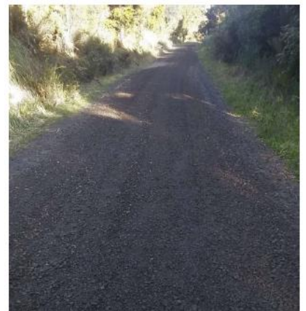
Duddy Rd – Maintenance Metalling
