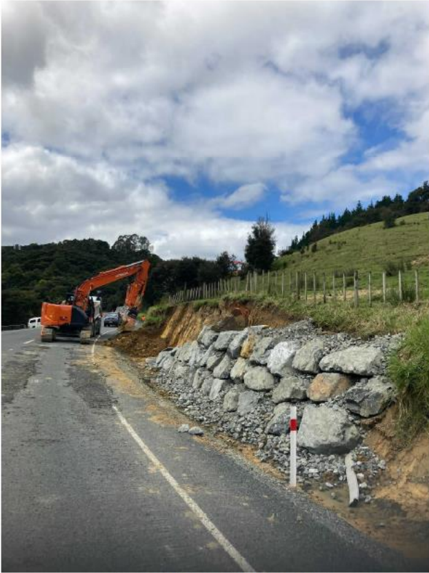
Figure 5: Peria Rd Seal Extension Slip Repairs
