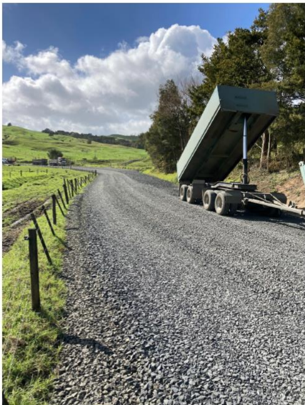
Figure 11: Pawarenga Rd Rehab Pavement Overlay
