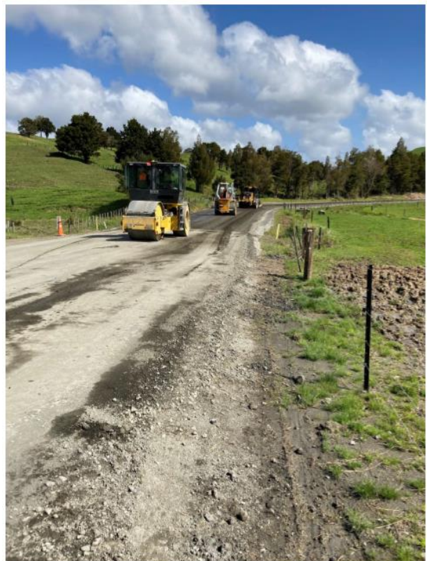
Figure 12: Pawarenga Rd Rehab Stabilising
