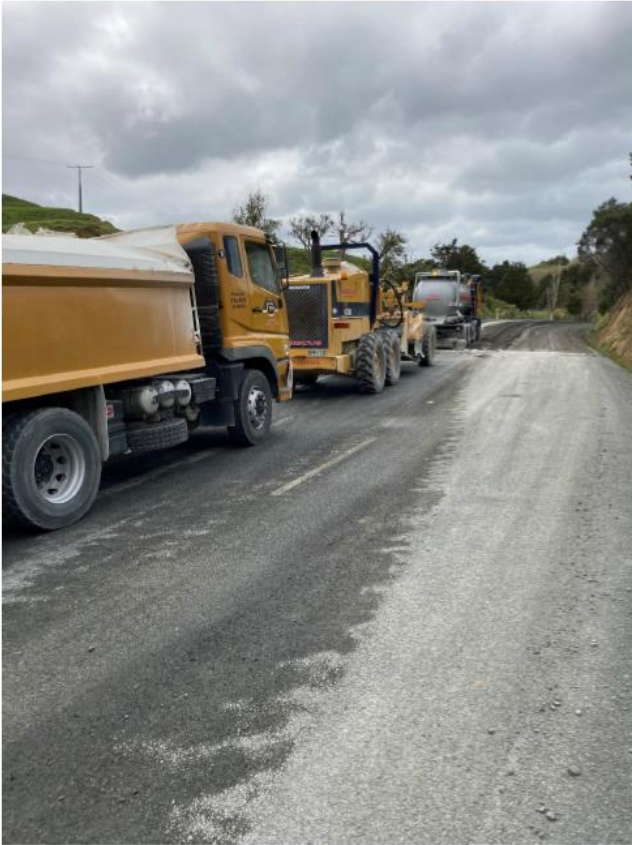
Figure 13: Pawarenga Rd Rehab Stabilising
