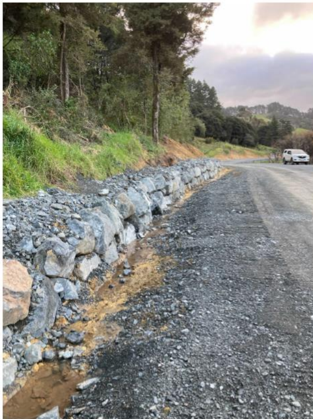
Figure 7: Peria Rd Seal Extension Toe Support
