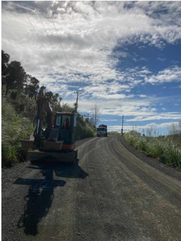
Figure 9: Parapara Rd Testpits prior to overlay
