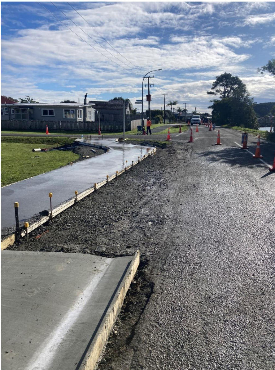
Oruru Road New Footpath Construction
