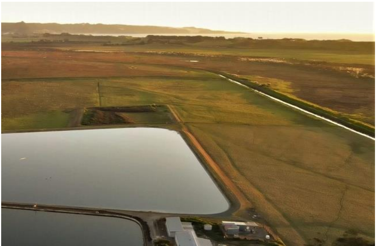
Figure 18 Sludge storage facility and Waihoe Channel (2021)
