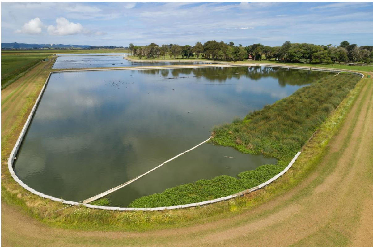
Figure 16 Kaitia WWTP constructed wetlands (2021)
